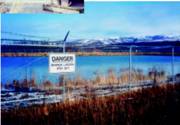
Sewage Lagoons are a typical wastewater treatment option.
