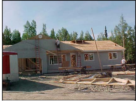
Residential construction in Territory 1.
