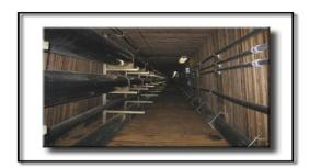
The Utilidor supplies water to fire hydrants throughout the town. Hydrants are "dry barrel", meaning, no water is actually in them until an internal stem is driven down to open them up. The water in this system is constantly circulating."
