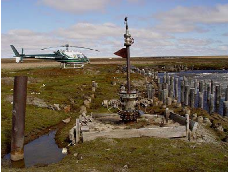
Awuna wellhead with exposed wooden pilings and Styrofoam.
