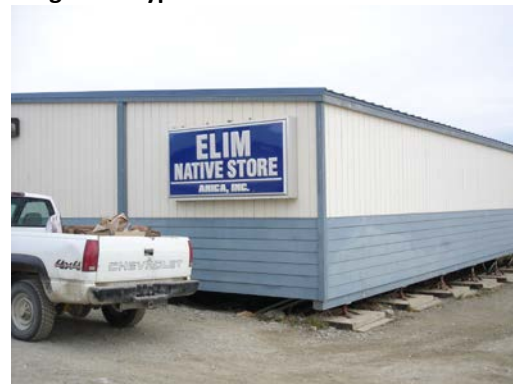
Figure 2. Typical Post-and-Pad Foundation
