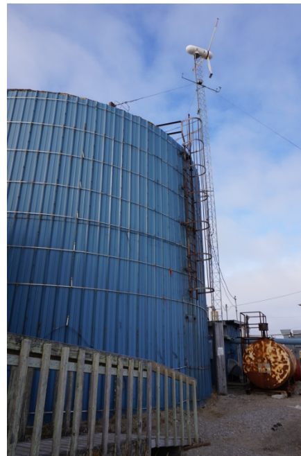
Water Storage Tank
