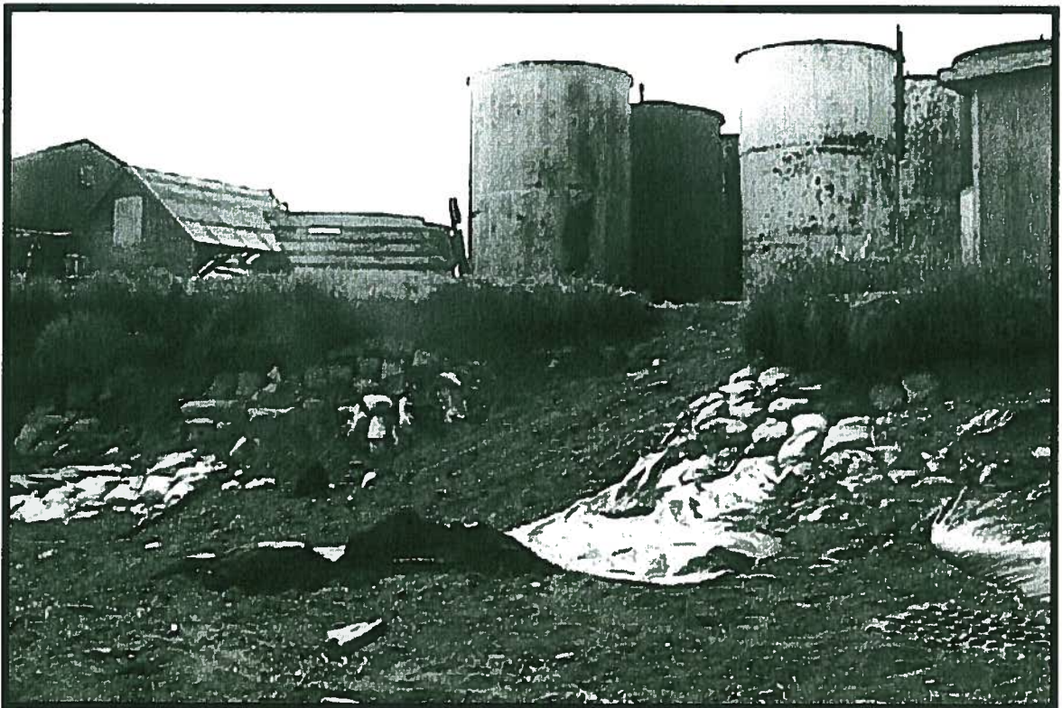
Photo 14: Kivalina. Beach erosion on lagoon side. Note sandbags used to slow erosion. Unknown photo date. 2003 +
