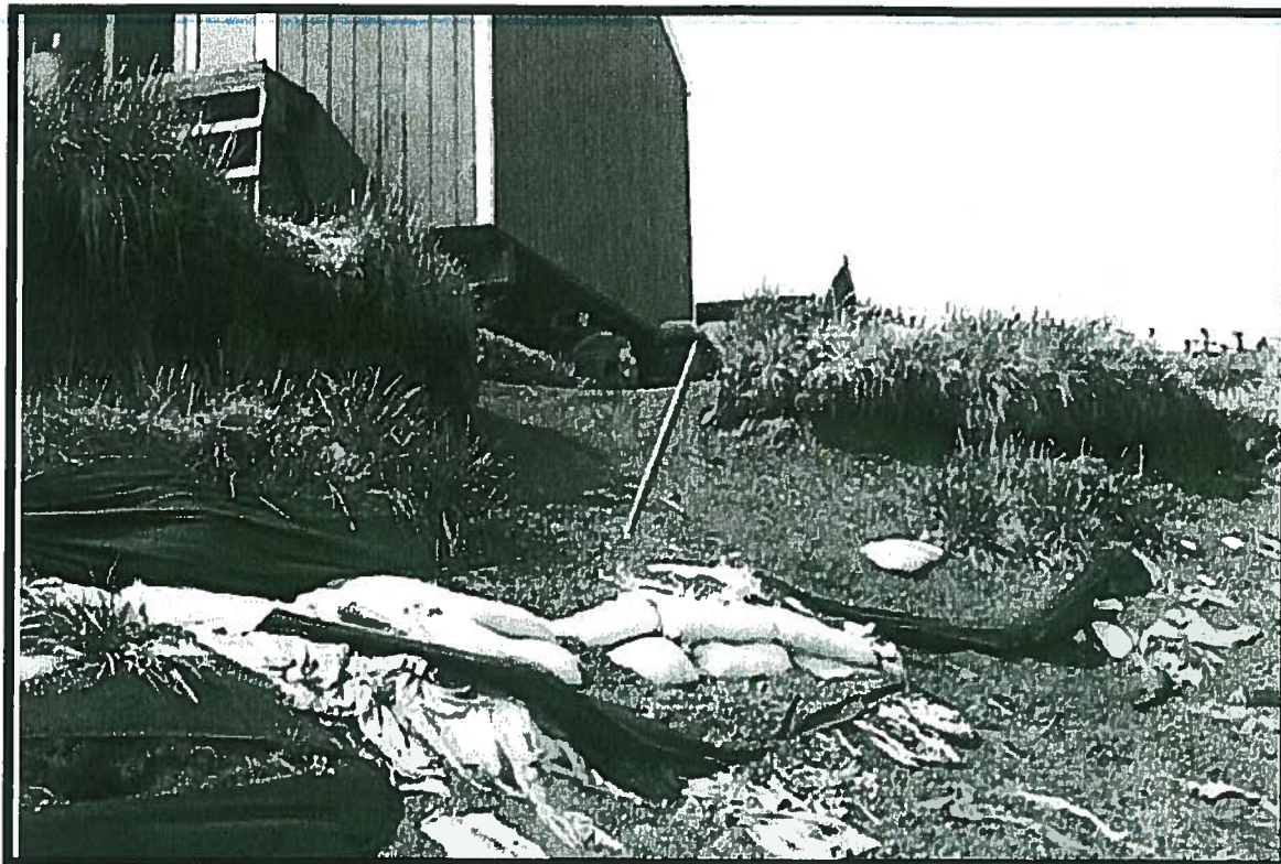
Photo 9: Kivalina. House on lagoon-side being undermined by erosion. Unknown photo date.
