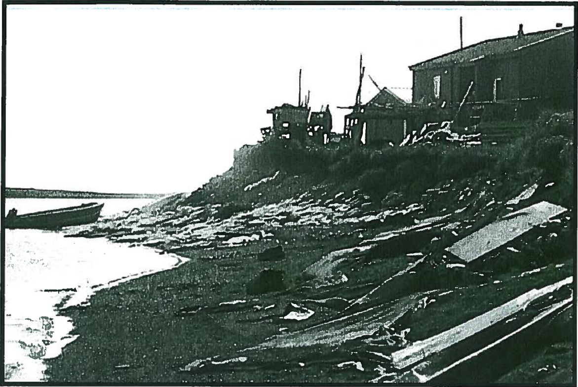
Photo 13: Kivalina. Beach erosion on lagoon side. Note sandbags used to slow erosion. Unknown photo date. 2002 2003 +
