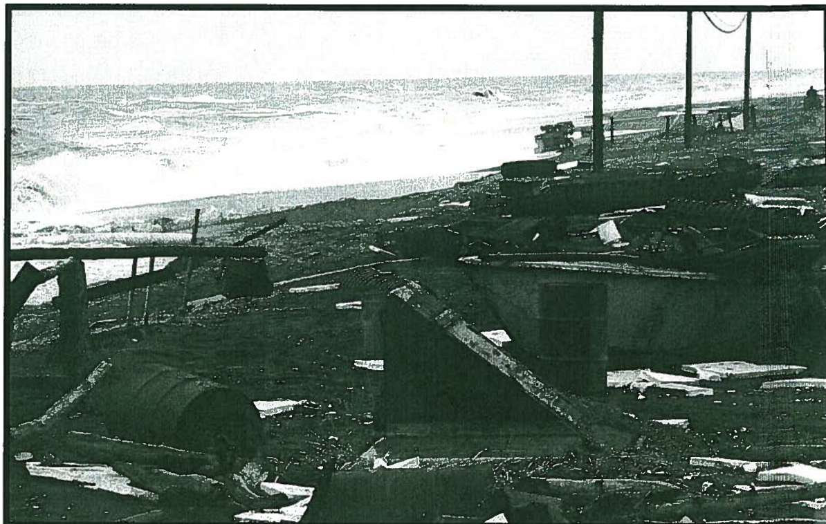
Photo 16: Kivalina. Storm surge causing erosion. Note sewer outfall pipe exposed, sewage leach field has been destroyed. The power poles seen here have since been destroyed by storm surge erosion. Photo date May 31, 2004.
