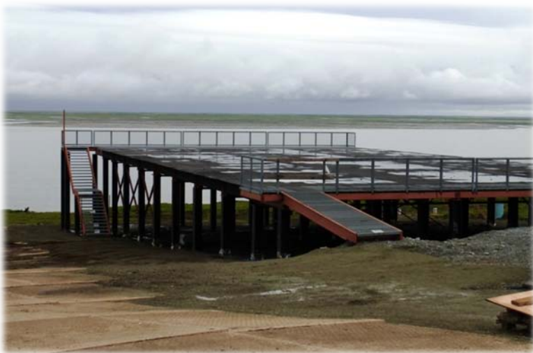
Foundation for Evacuation Center
