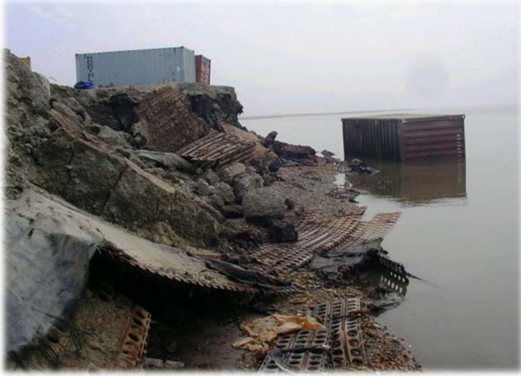
Barge Landing Destroyed in 2005
