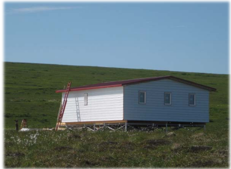
Home #7 Constructed in 2016
