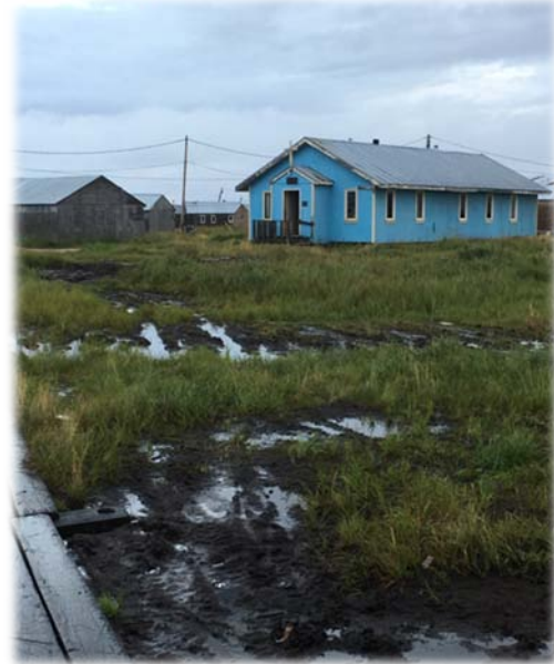
Subsiding Ground Around Newtok Church
