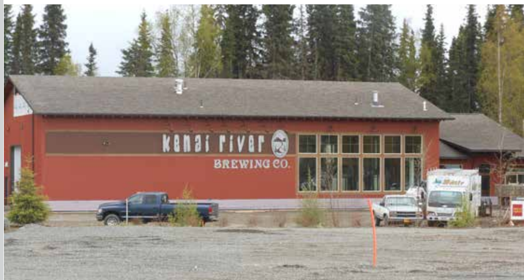
A new building at the Kenai River Brewing Co., a successful brewery in the region
