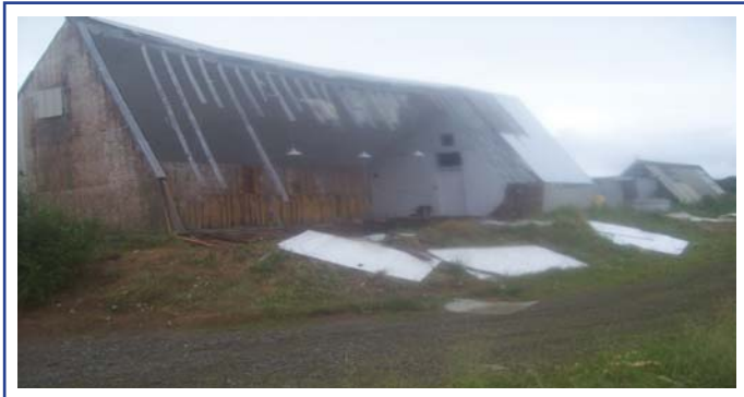
Large greenhouse being demolished due to unsafe roof
