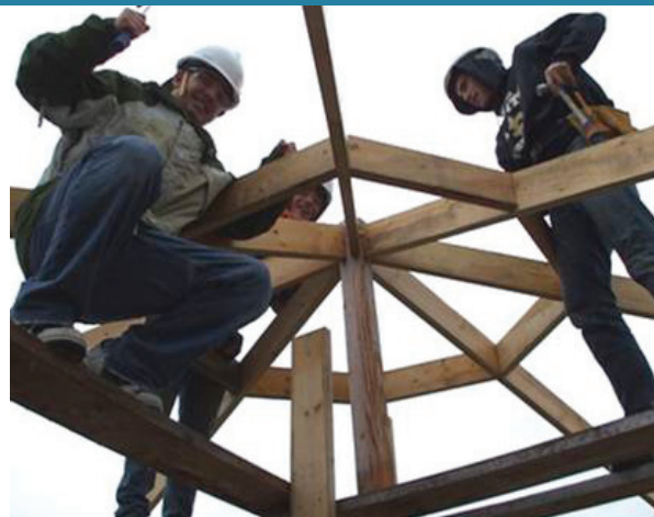
Kenai Peninsula Construction Academy students build a greenhouse. Photo courtesy of KPEDD.
