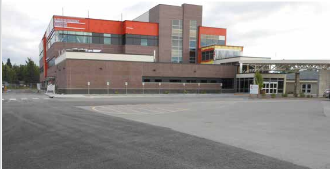
New Central Peninsula Hospital outpatient services building
