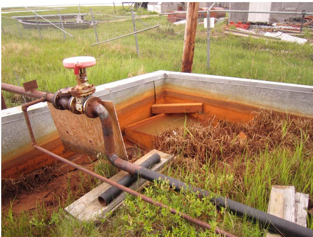
Photo 12: Rust staining in SE corner
