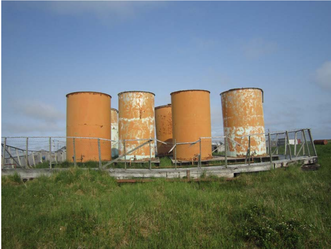
Photo 15: Fencing in disrepair, wood platforms subsiding
