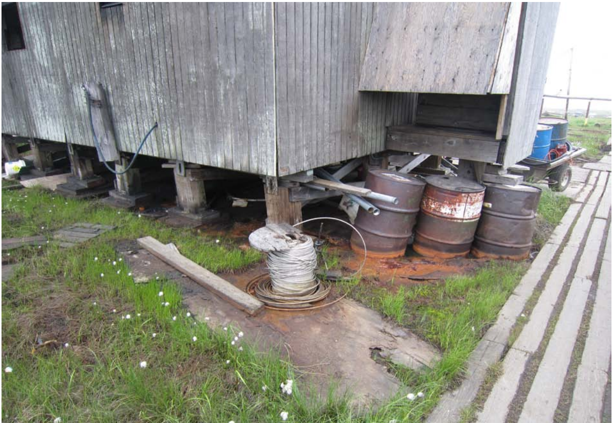
Photo 27: Significant oil staining below building.
