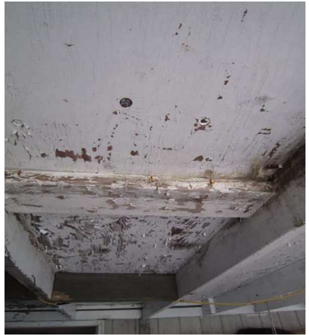
Photo 31: Peeling paint may be lead containing or lead based.
