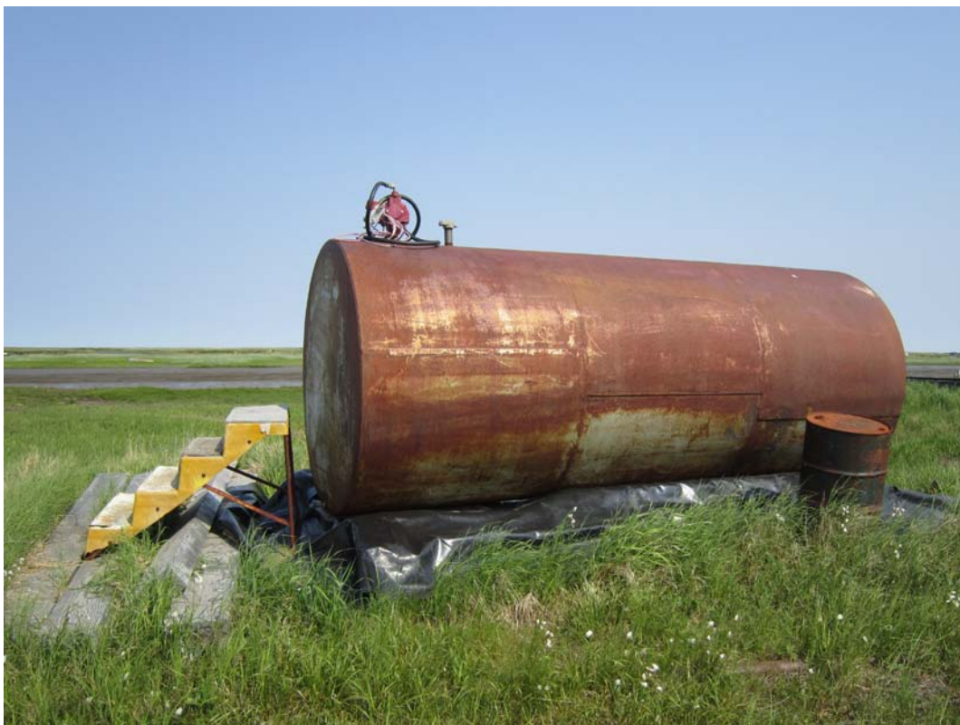
Photo 22: 3000 gallon tank, in use, no secondary containment
