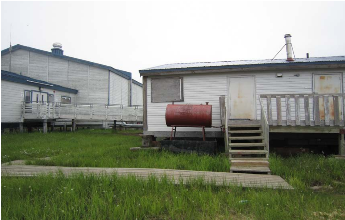
Photo 13: 250 gallon tank with metal container box below.
