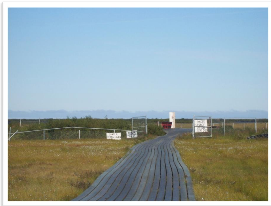
Photo 28: Fencing around sewage lagoon slumps as land subsides.
