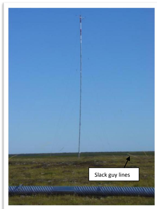
Photo 10: Tower located between sewage lagoon boardwalk and runway. Note the slack in the guy lines.
