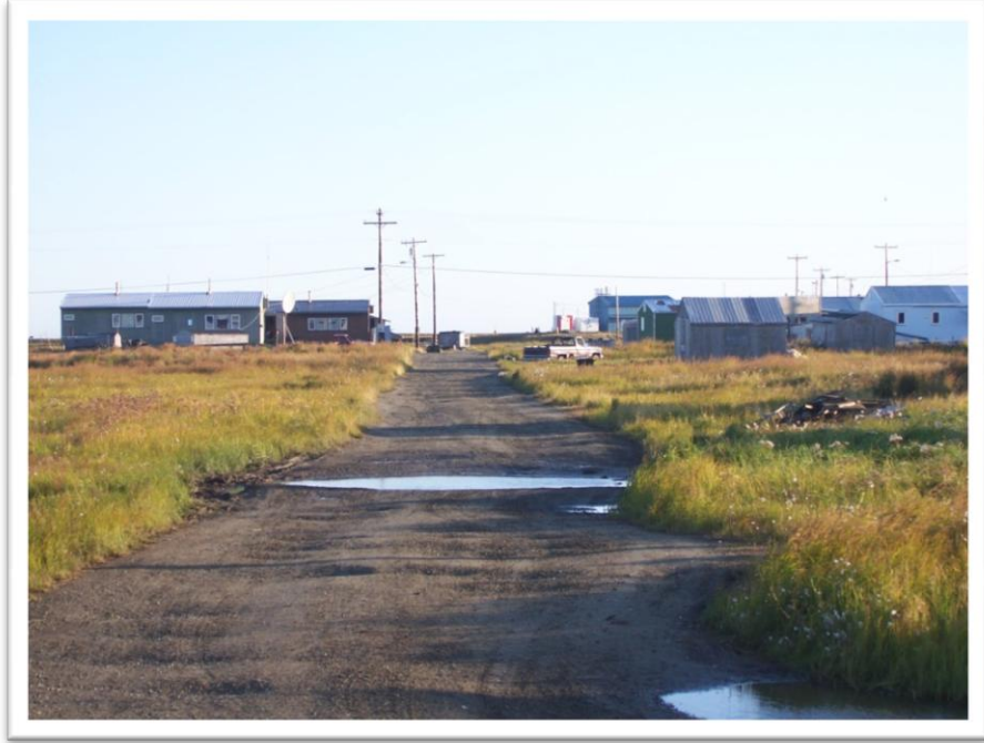
Photo 33: Ponding in gravel road from airport through town.
