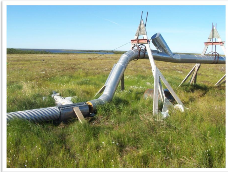
Photo 27: Sewer pipe to sewage lagoon northwest of town.
