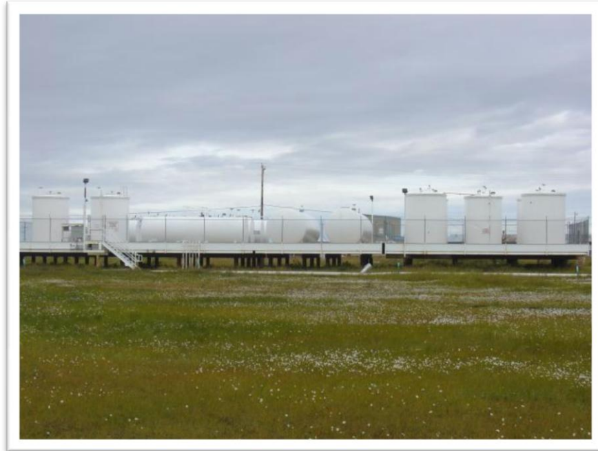
Photo 11: Pile support fuel storage facility.
