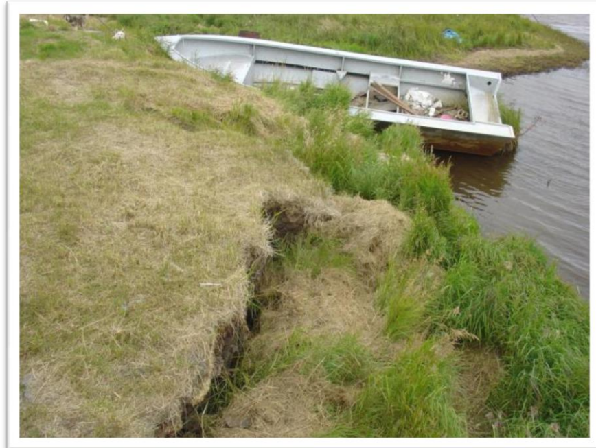
Photo 21: Riverbank erosion. The grass mat likely reduces the rate of erosion, as it provides some insulation against thaw and resistance to water flow and wake erosion.
