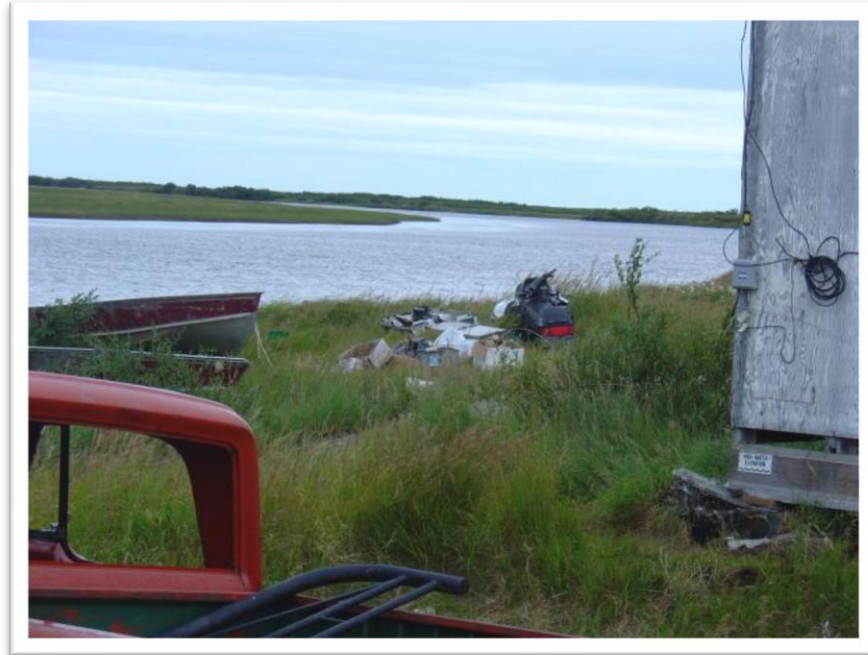
Photo 17: Proximity of house to Pitmiktakik River at south end of Atmautluak. Note high water elevation mark on structure.
