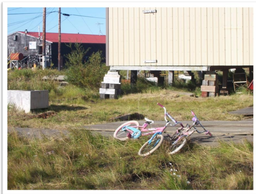
Photo 32: Blocks level and support school building.
