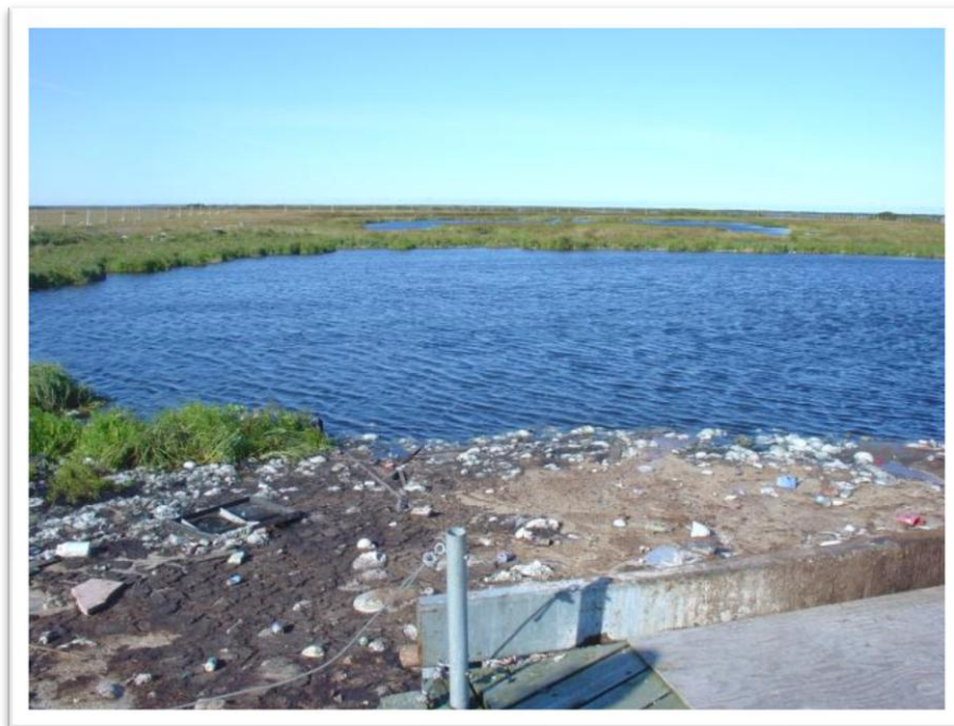
Photo 16: Primary wastewater treatment lagoon located approximately one-half mile northwest of the main body of the village.
