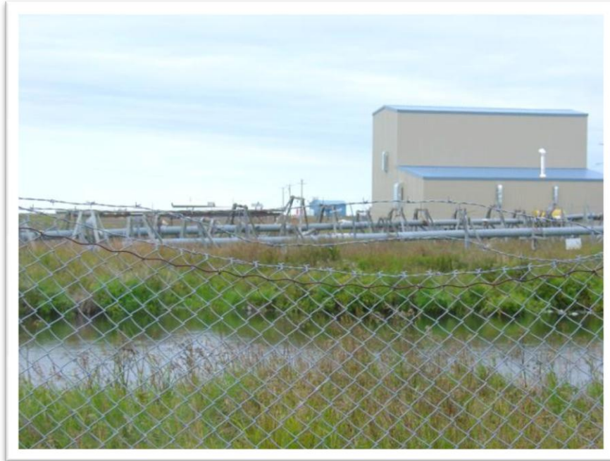
Photo 15: Old wastewater treatment lagoon in central part of town. New school wastewater treatment plant in background.
