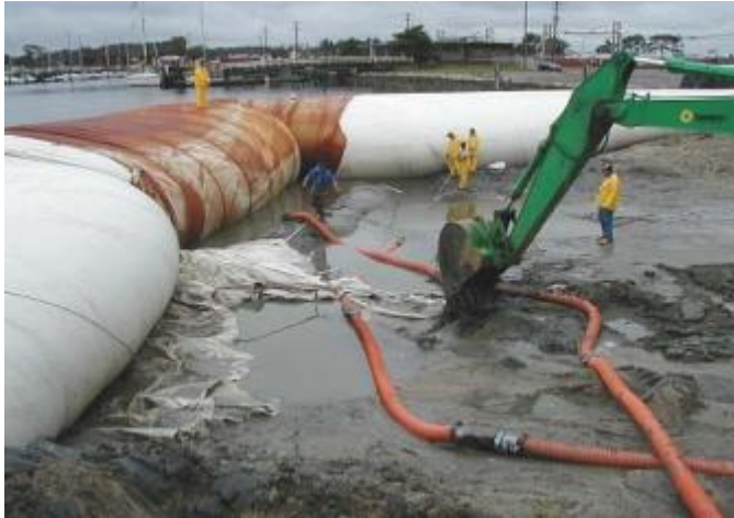
Figure 13: Temporary Cofferd Dam
