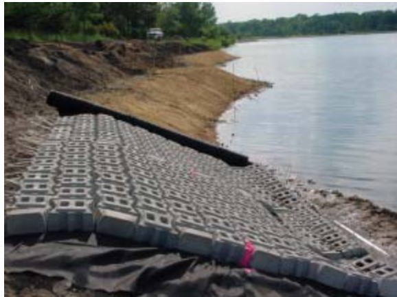
Figure 9: Examples of ACB Installations. The right photo shows the revegetated ACB installation at Nunapitchuk.
