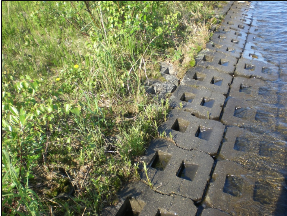
Figure 13. ACB installation at Lake Hood/Spenard Lake channel, Anchorage, AK.
