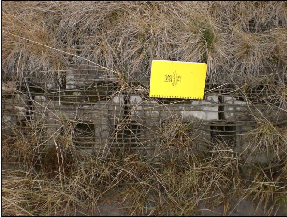
Figure 11. ACB at Nunapitchuk Airport embankment along Nunavakanukakslak River.
