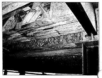
Above: Discoloration of structural joist members by water infiltration through the decking.
