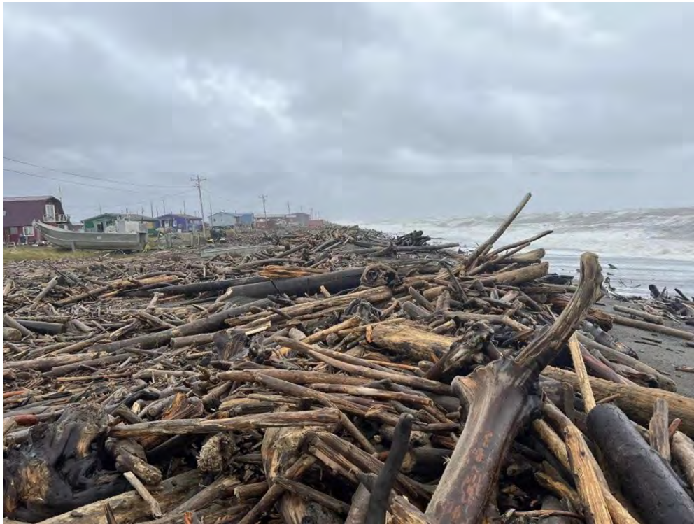
Figure 10. Shaktoolik's berm destroyed in the storm
