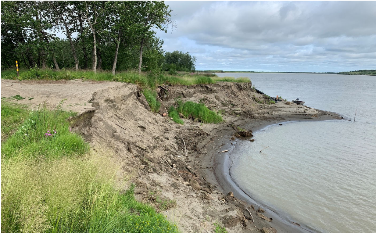
Figure 4: Bank erosion in front of structures #600-602.
