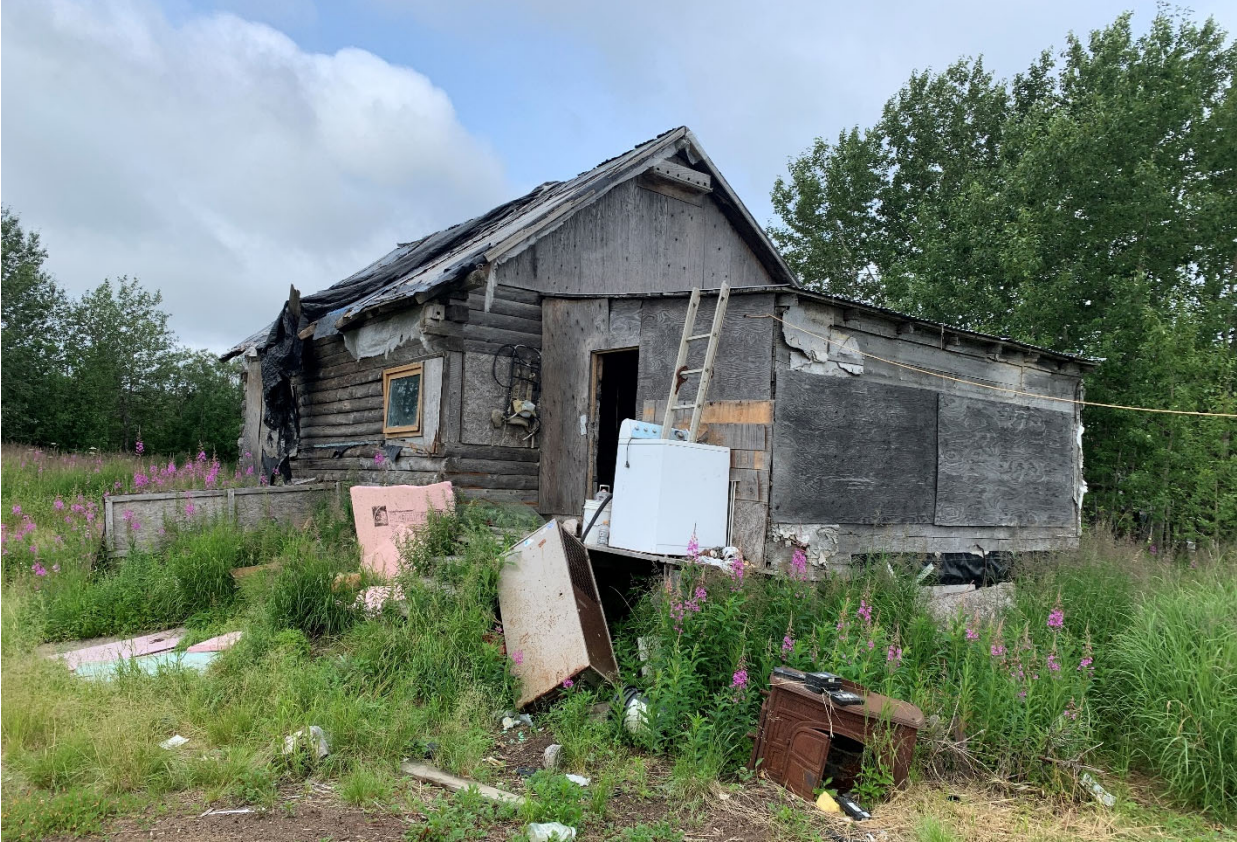
Figure 3: Abandoned Structure #602 identified for demolition and removal.
