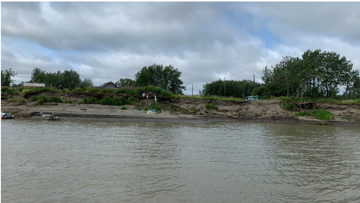
Figure 5: Bank erosion in front of structures #600 - 602 as seen from the Kuskokwim River.
