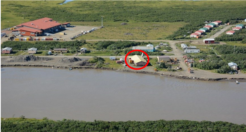
Figure 2: The Tribal Hall (circled in red) is critical infrastructure in Alakanuk, Alaska and threatened by erosion. It is a top community priority to relocate the building to a safe location within the community. Source: Alaska ShoreZone.
