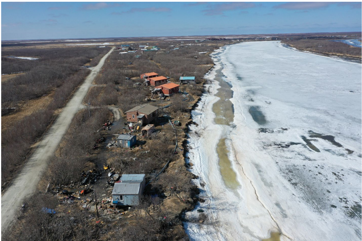
Figure 9: Aerial image of the most imminently threatened homes in Alakanuk. The home in figure 8 is located on the top of the image with a blue roof. Source: Village of Alakanuk.
