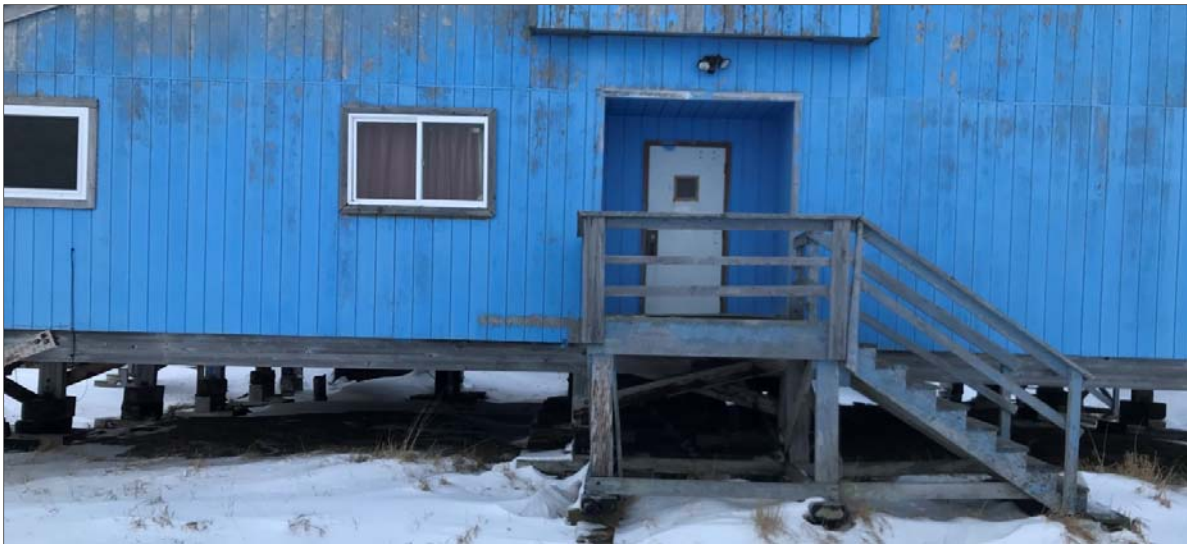
Figure 9. Head Start Building - Shifting Towards River Bank
