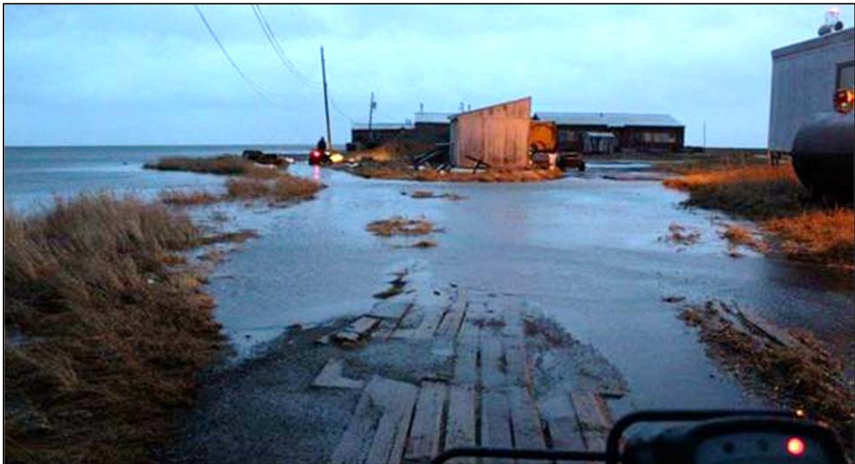
Figure 7. Head Start building access, morning October 5, 2017.
