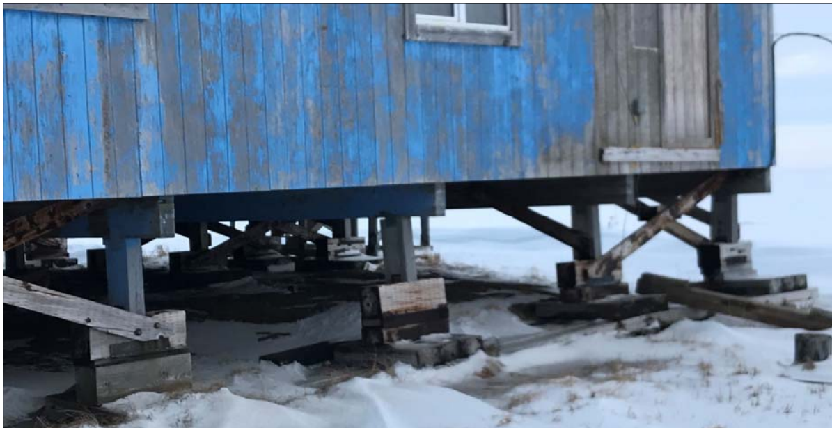
Figure 8. Head Start Building Foundation
