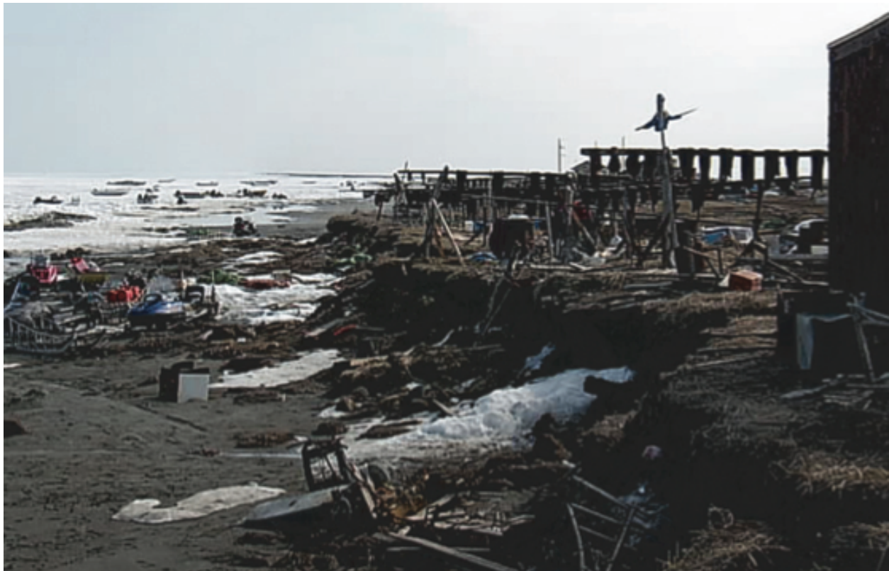
Figure 1: Sea Erosion at Shishmaref June 2003 (Source: GAO)
