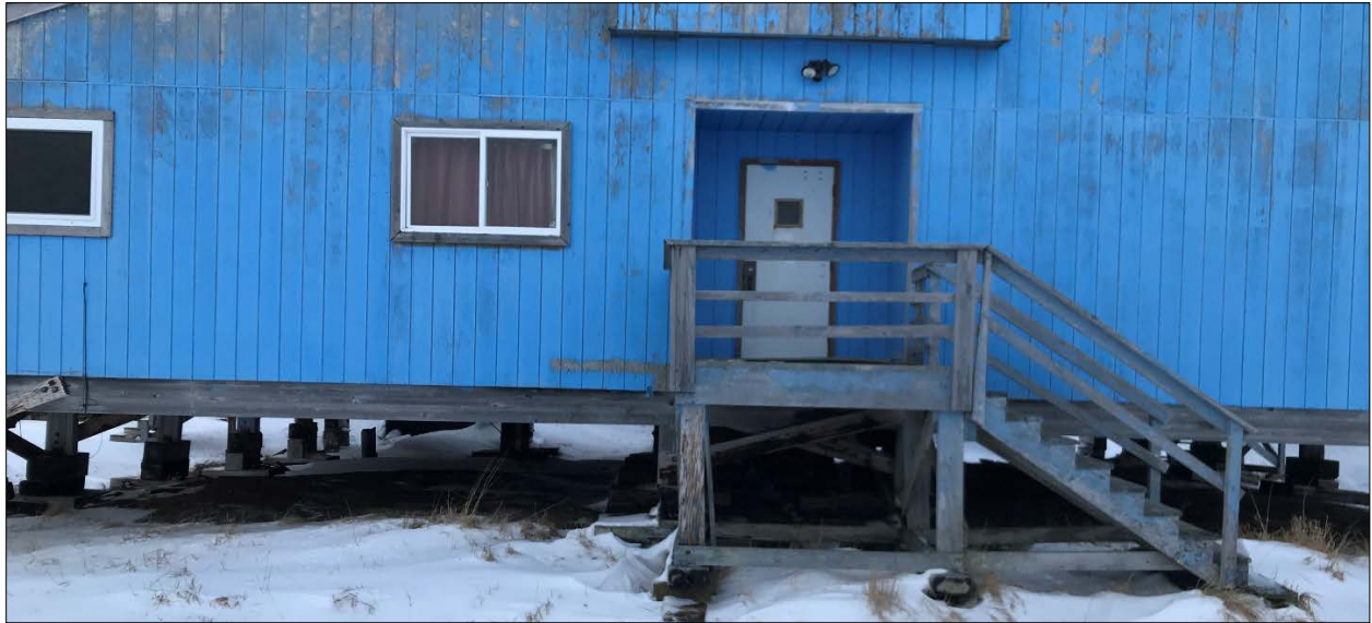
Figure 13. Head Start Building - Shifting Towards River Bank
