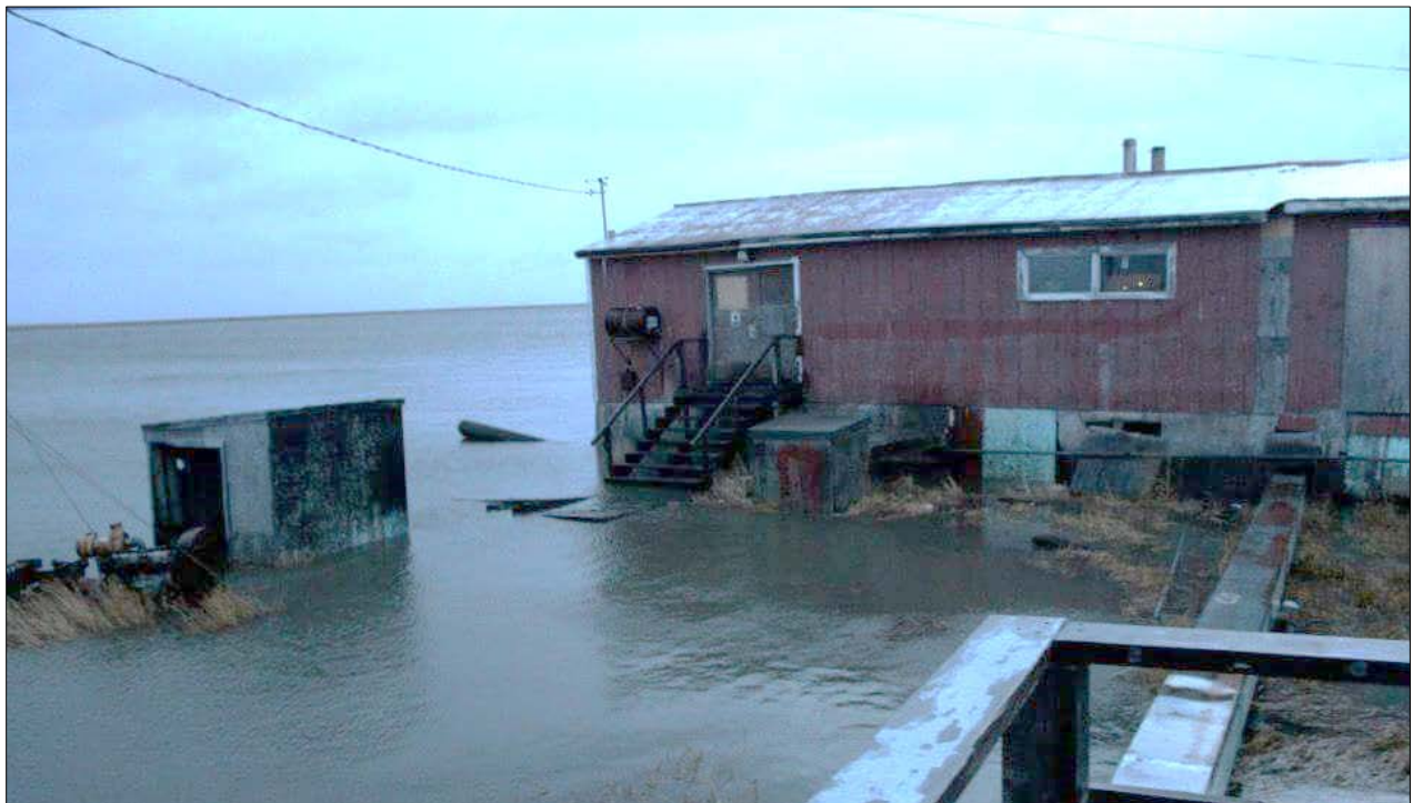
Figure 14. Head Start Utility building as seen from the entrance to the Head Start building.
