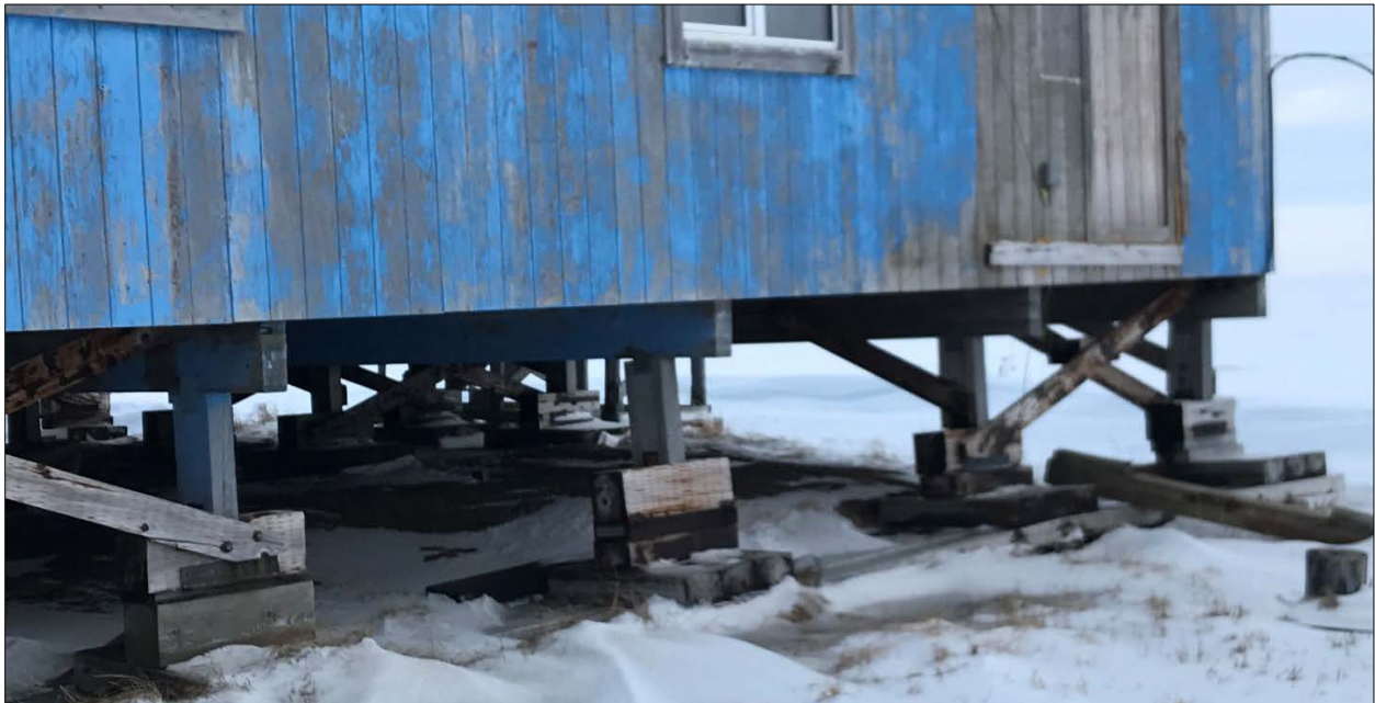
Figure 12. Head Start Building Foundation
