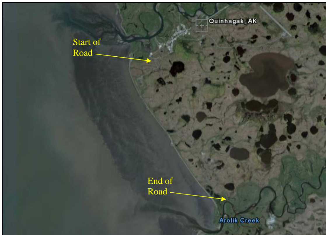
Figure 6.6.3: Aerial view (©Google Earth) of the existing road to Arolik Creek. Note: Development of this alternate landing site would require further study to determine accessibility.
