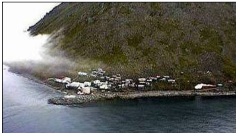
Figure 6.2.2: The landing areas at Diomedede on either side of the breakwater.
