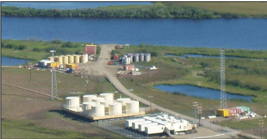
Figure 6.11.2: The main barge landing and staging area at Selawik.
