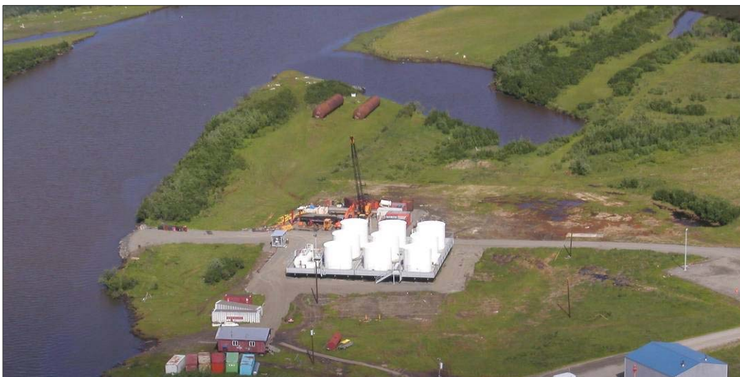
Figure 6.3.3: The landing and staging areas at Kotlik.
