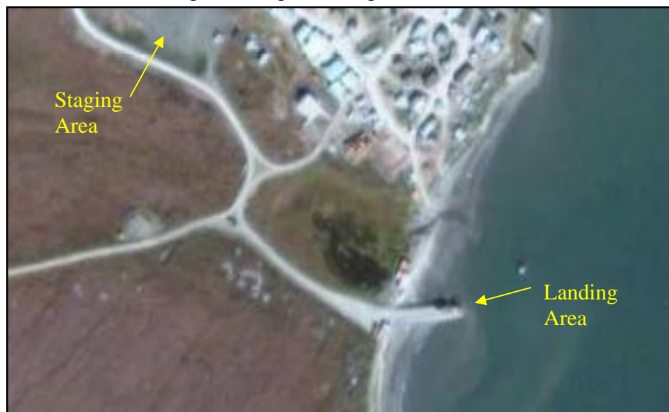
Figure 6.6.9: Former gravel/rock causeway at the barge landing site at Toksook Bay (©Google Earth)
