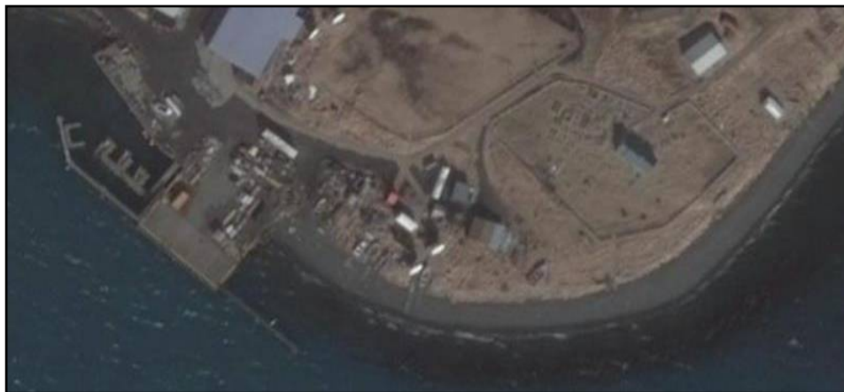
Figure 6.13.2: Aerial view of the Akutan dock (©Google Earth).
