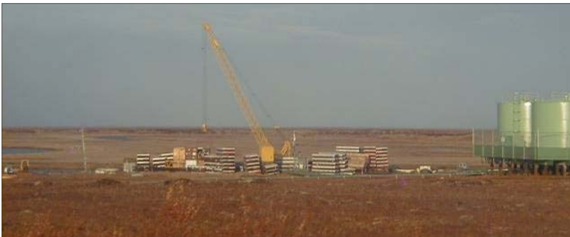
Figure 6.6.4: Kongiganak, the staging area at the main barge landing site.
