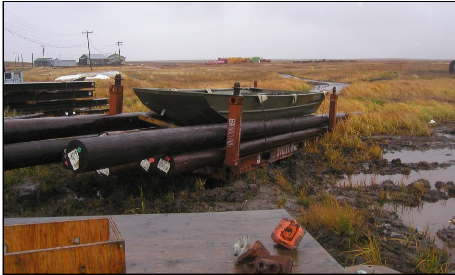
Figure 6.6.5: The Kongiganak staging area is often wet, cargo sinks into ground.
