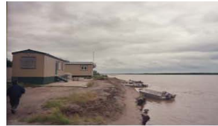
Yukon Rv Shoreline Erosion 3.JPG
