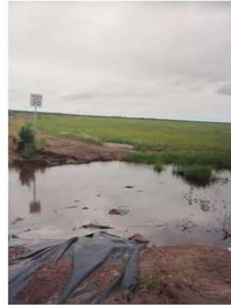
Airport Access Road Damaged from Flooding 3.JPG
