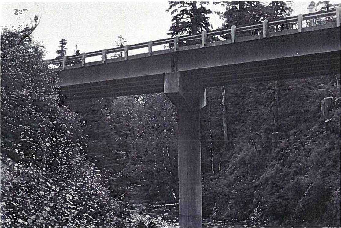
FIGURE 2 - The new North Tongass Highway Bridge spanning Whipple Creek.
