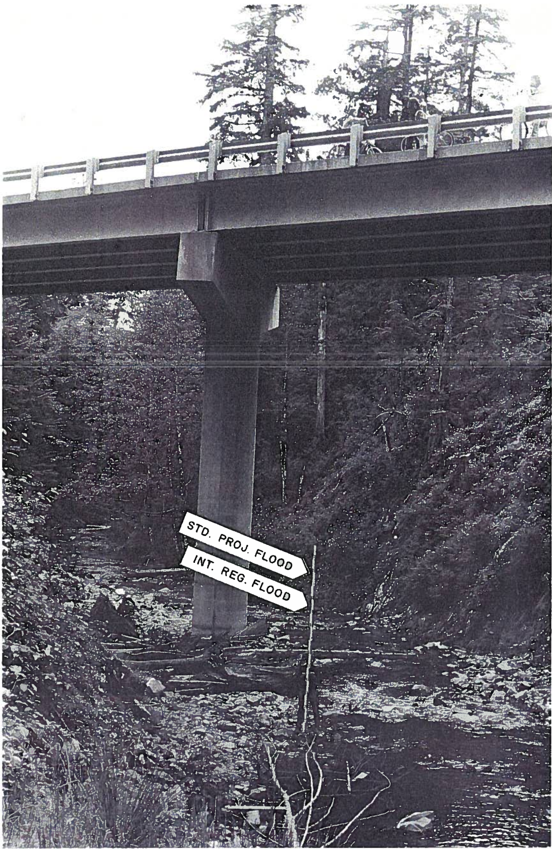
FIGURE 5 - Future flood heights at upstream side of the new North Tongass Highway Bridge.
