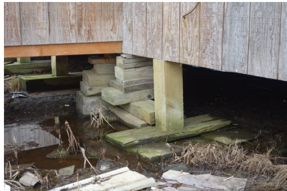
Figure14: Residence Footing on Undrained Soil
