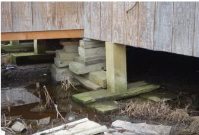
Figure10: Footing on Undrained Soil
