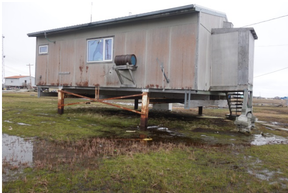
Figure13: Pile Supported Residence
