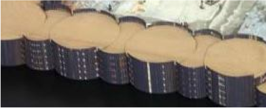
Figure 27: Circular Sheet Pile Wall System
