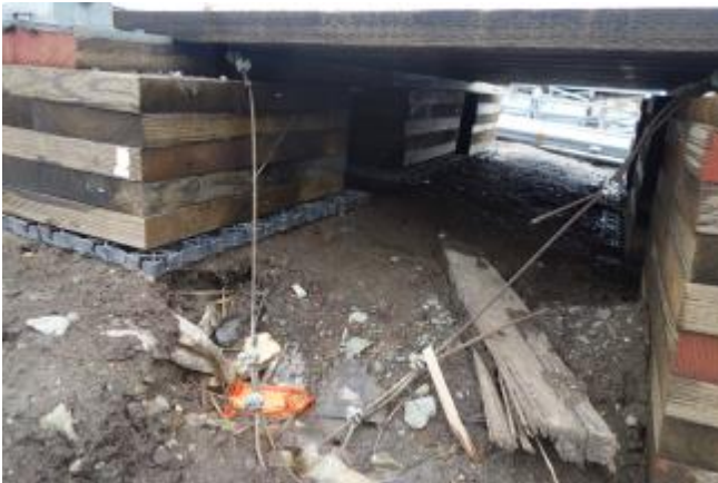
Figure 16: Boardwalk Footing Placed on Well Drained Soil
