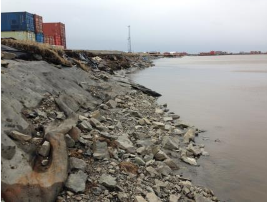
Figure 22: Riprap In Disrepair, Reach 2
