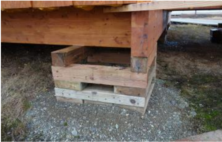
Figure 13: Foundation Pad on Perched Ground
