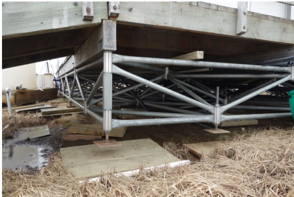
Figure 10: Halibut Plant, Unsupported Legs
