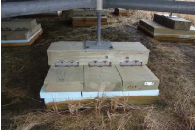
Figure 15: Insulation Between Timber Pads
