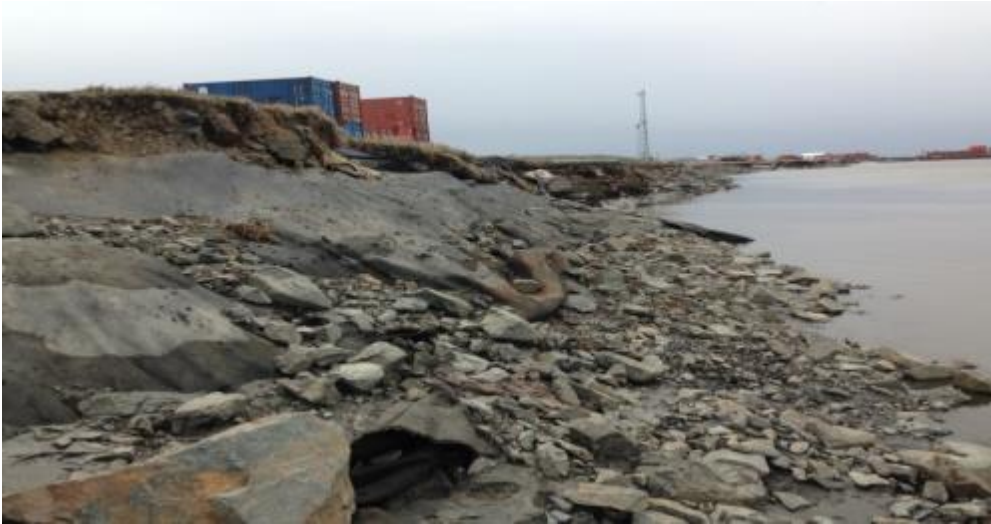
Figure 6: Existing Riprap Revetment Reach 2
