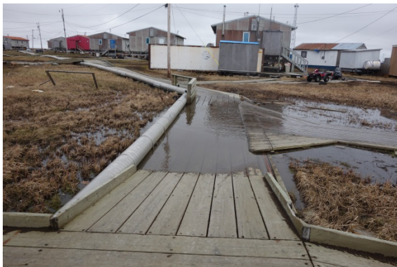
Figure 7: Boardwalk in Ponding Water
