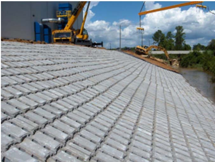
Figure 19: Articulating Concrete Blocks
