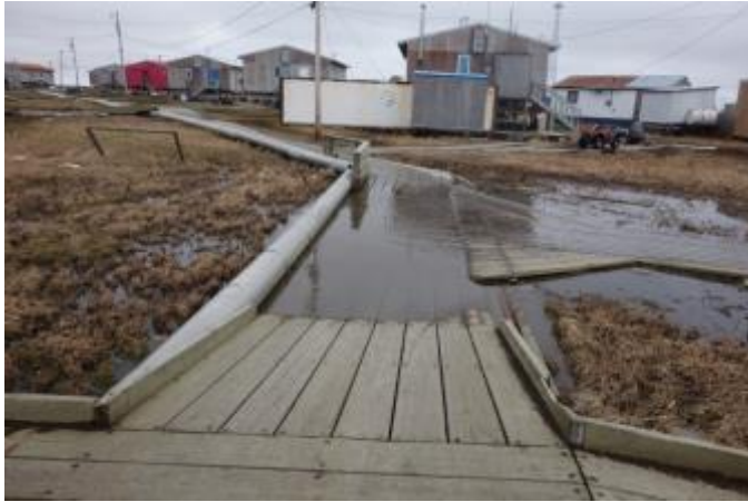
Figure11: Boardwalk Settlement, Low Wet Area
