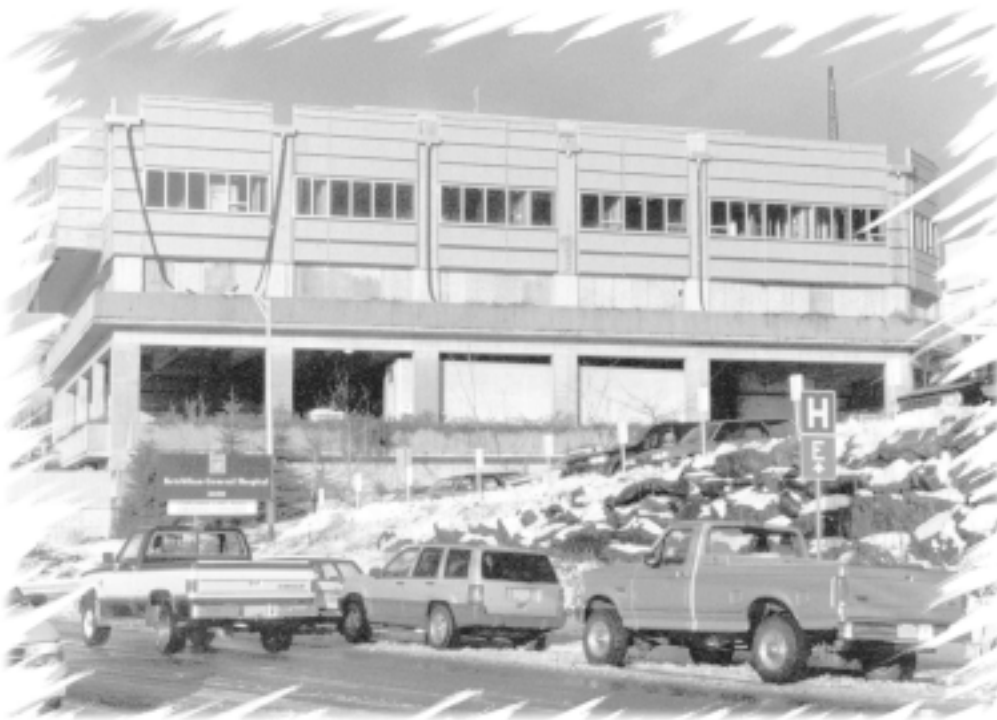
New construction at the City-owned Ketchikan General Hospital
