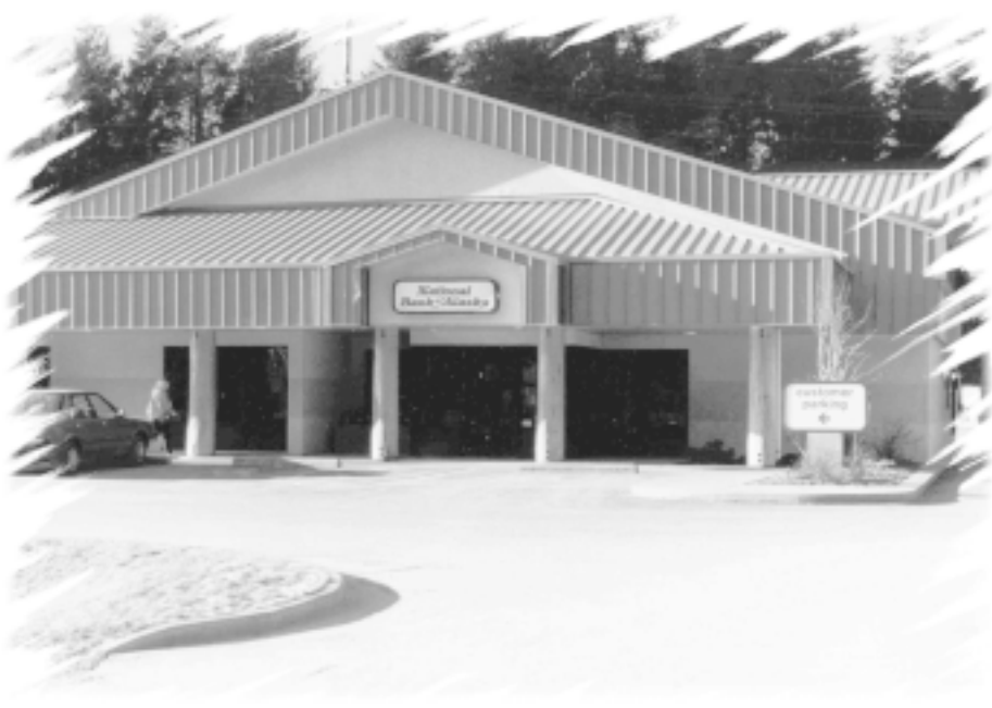
National Bank of Alaska branch located in the area proposed for annexation
