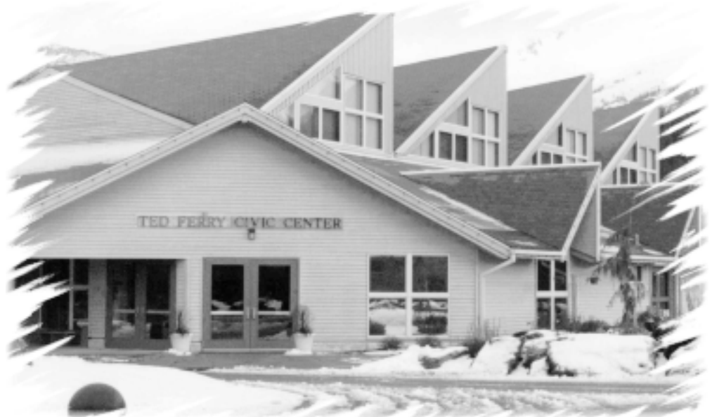
Ted Ferry Civic Center in Ketchikan, one of the City facilities serving the entire community
