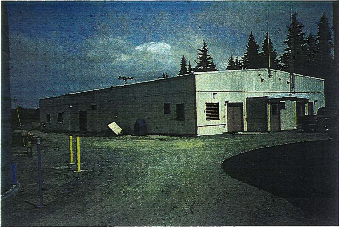
City of Homer: Water Treatment Plant
