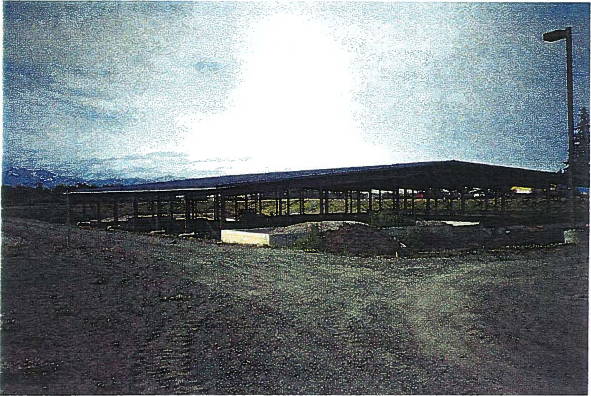
City of Homer: Drying Bed Structure
