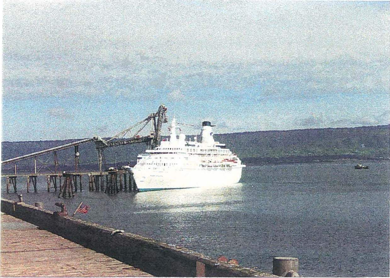
City of Homer: Deep Water Cargo Dock
