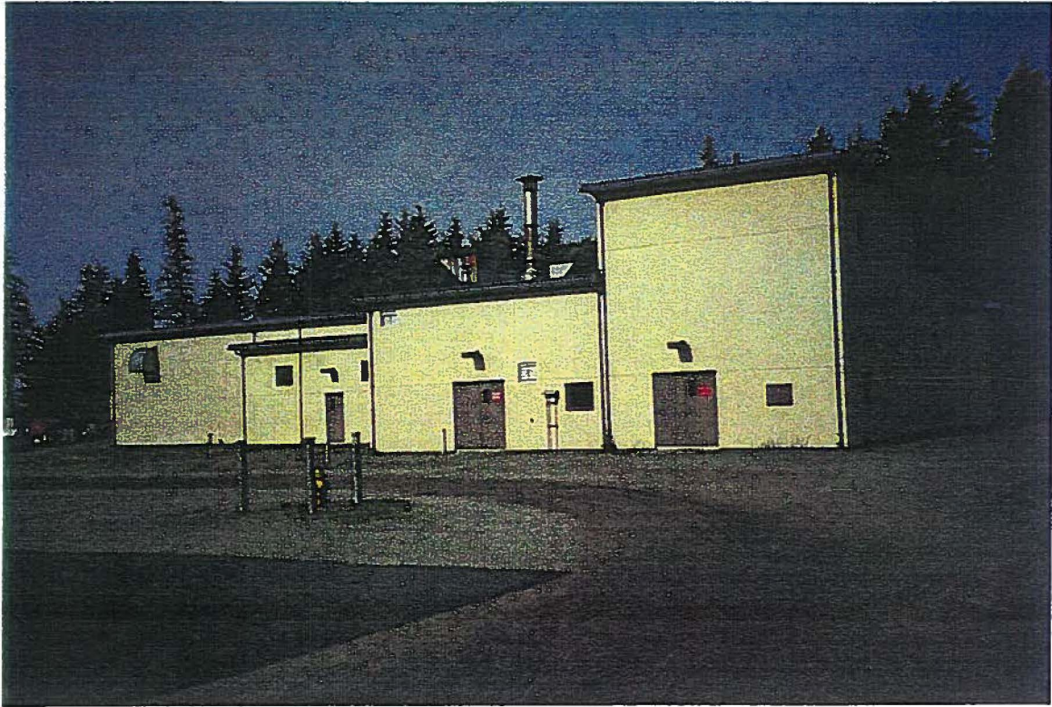
City of Homer: Sewer Treatment Plant
