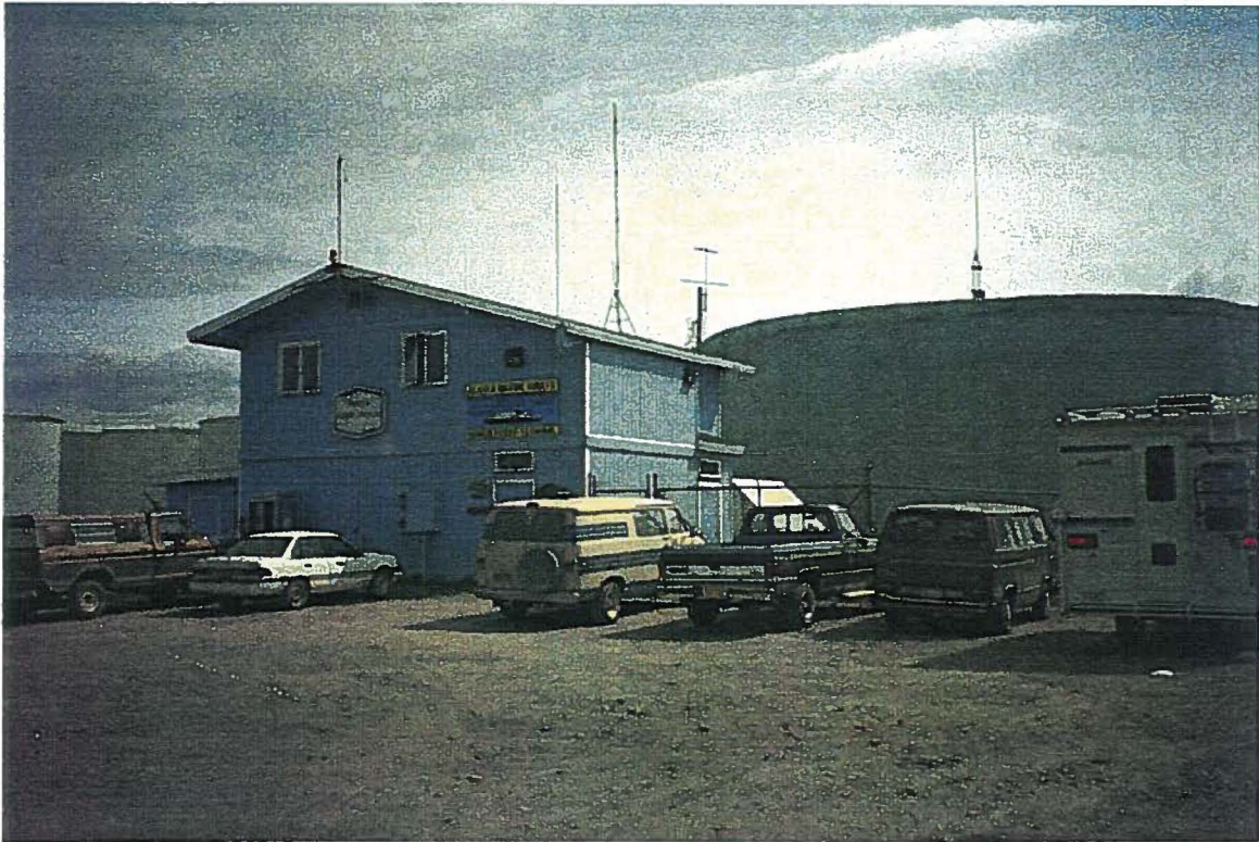
City of Homer: Ferry Office/Pump Station
