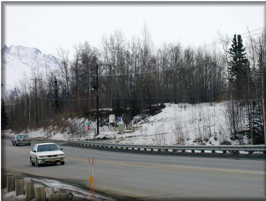
Area H-Southside Palmer-Wasilla Highway.
