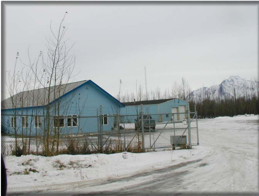
City of Palmer public works.
