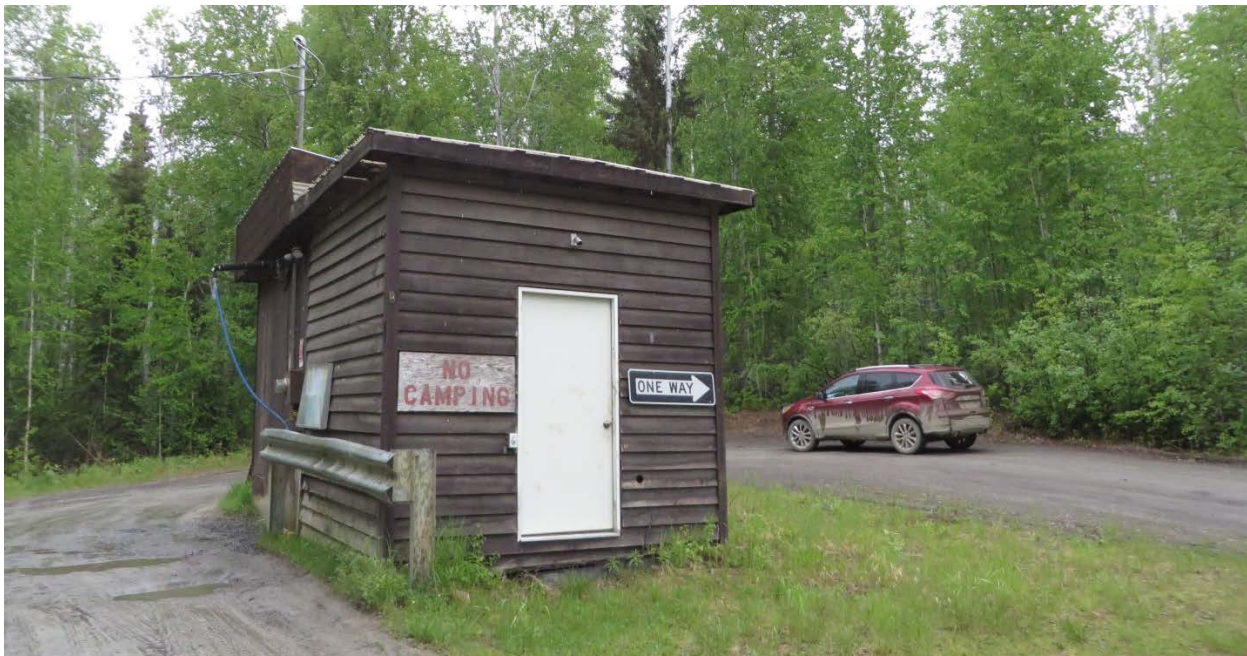
The community well house in Manley Hot Springs provides drinking water for residents, 2016
