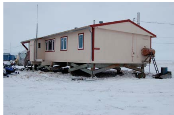
Above: piles create more surface area and heat loss
