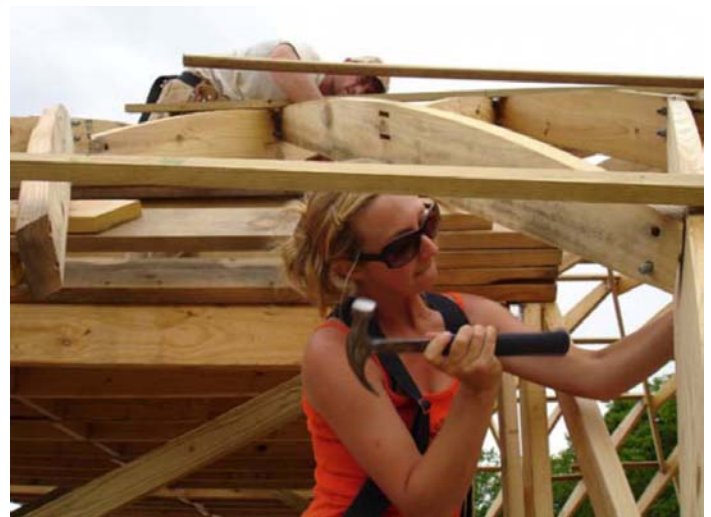
Above and Below: Lamella roofs are commonly constructed using unskilled and volunteer labor
