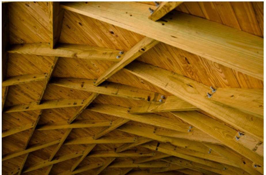
Below: interior aesthetic of lamella roof structure
