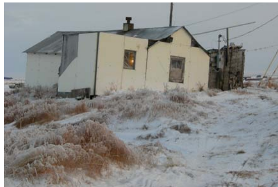
Above and Below: Thaw-bulb action
