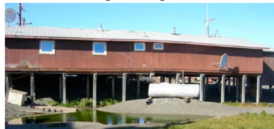
Piles can create subsidence issues
