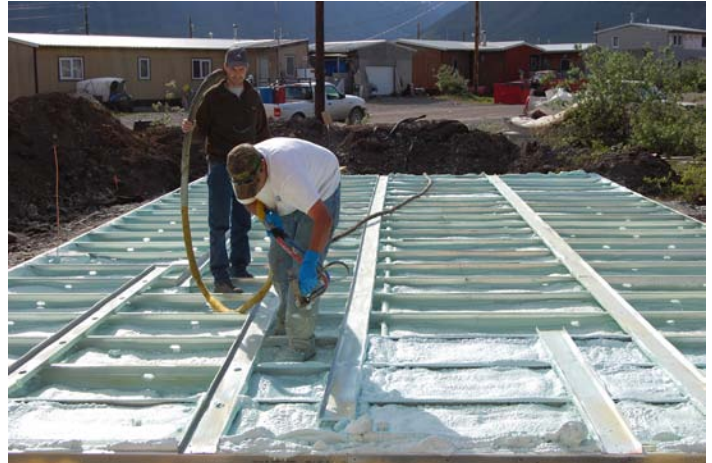
Above: An applicator sprays the floor in a residence in rural Alaska
