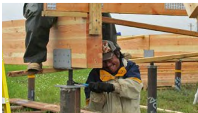
Figure 17. Adjusting foundation screw jacks in Atmutluak, Alaska. (CCHRC Inc.)
