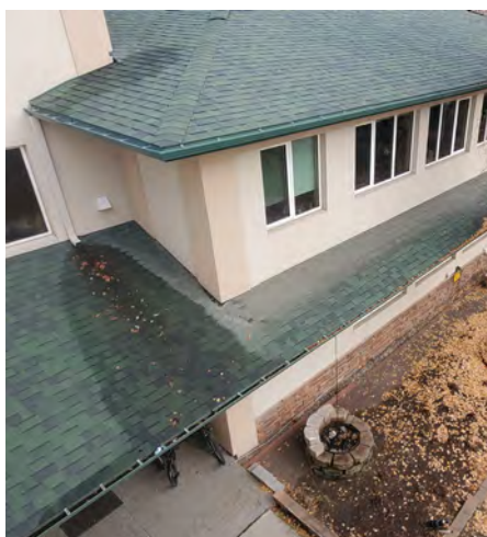
Figure 24: (left) Gutters and a downspout help direct rain and snow-melt. (right) Drain spouts and flexible drain channels direct water away from the building and into a ditch that feeds a retention pond (in the distance). (G. Davis, NREL)
