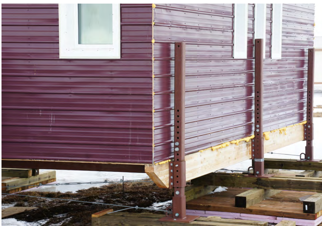
Figure 26. Adjustable foundation example. (B. Tracey, Point Lay)
