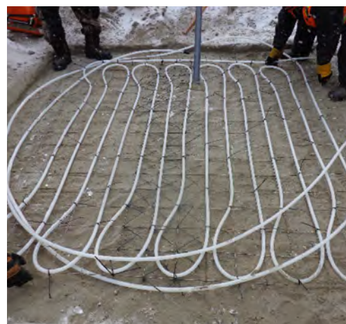
Figure 23. Active cooling loops laid under a slab on grade commercial foundation. (CCHRC Inc.)
