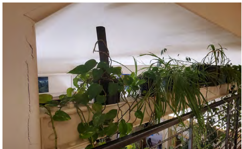
Figure 14. Cracks in drywall caused by ground movement. (G. Davis, NREL)
