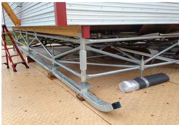
Figure 22. Mertarvik skidded space frame. (CCHRC Inc.)
