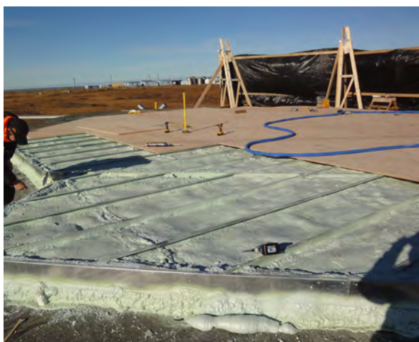
Figure 20. (Top and right) Anaktuvuk floating raft foundation; (left) Quinhagak raft foundation under construction. (CCHRC Inc.)
