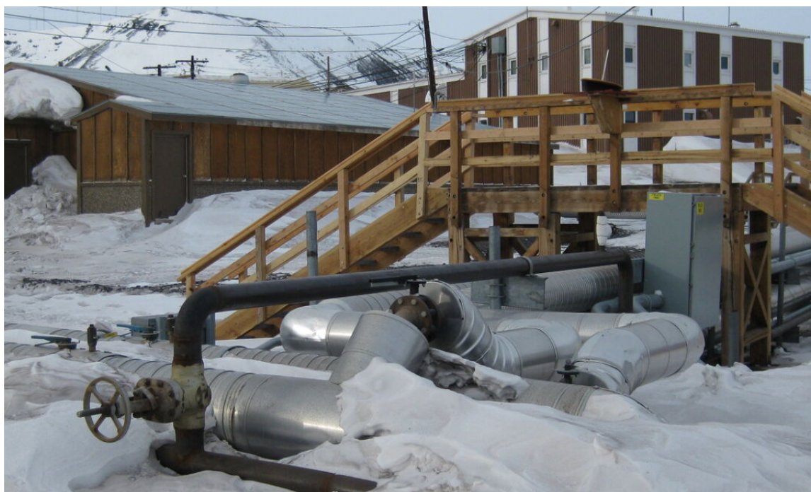
Figure 27. Insulated water and fuel pipes in Antarctica, further protected by a pedestrian bridge crossing. (Photo by G. Davis)
