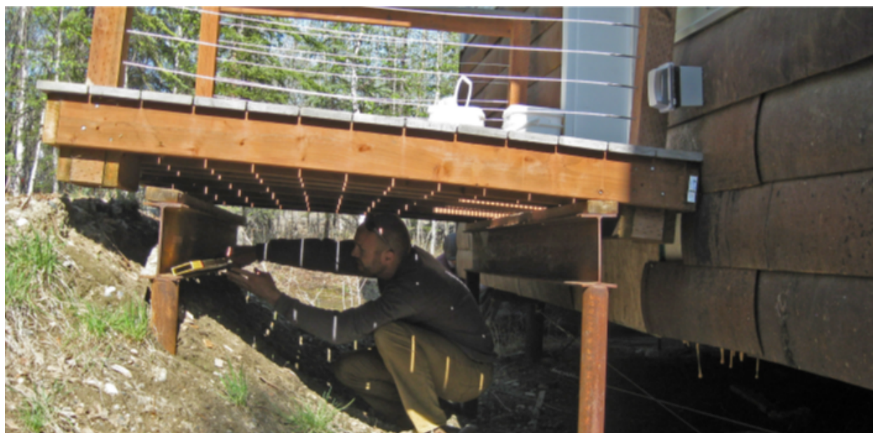
Figure 3: Example of frost jacking. (CCHRC Inc.)
