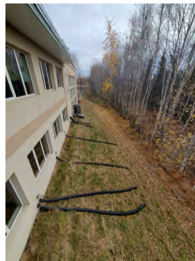
Figure 24: (left) Gutters and a downspout help direct rain and snow-melt. (right) Drain spouts and flexible drain channels direct water away from the building and into a ditch that feeds a retention pond (in the distance). (G. Davis, NREL)
