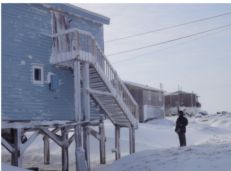
Figure 4: Ground subsidence. The stairs used to touch the ground. (M. Rettig, NREL)
