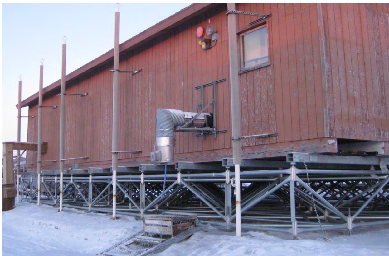
Figure 21. Space frame foundation with thermosiphons in Atmautluak. (CCHRC Inc.)
