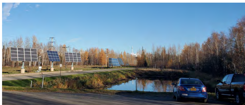
Figure 28. This meltwater retention pond is used by nearby buildings that channel rainfall and meltwater away from the building and parking area. (NREL)
