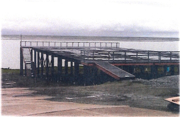
Foundation for Evacuation Center
