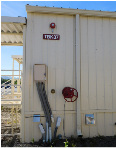
Sprinkler notification equipment
