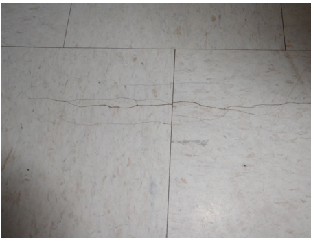
Cracking vinyl tile at module connection
