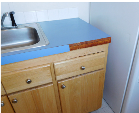
Damaged plastic laminate countertops
