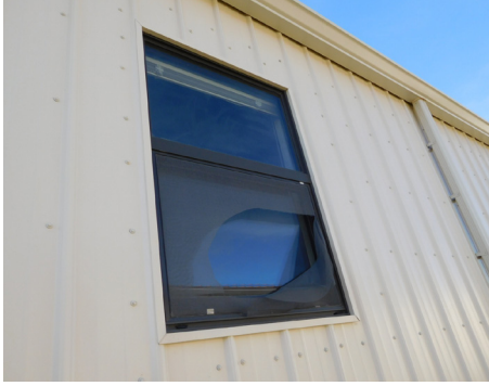
Damaged insect window screen
