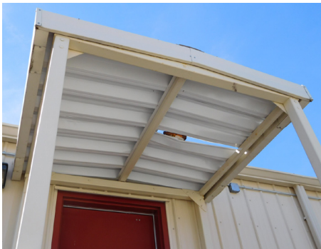
Damaged steel entrance canopy
