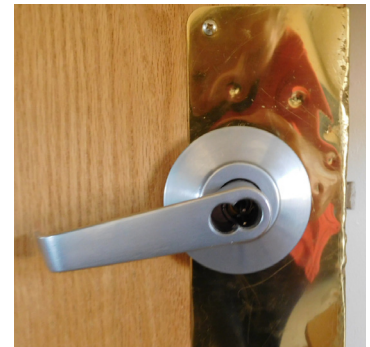
Damaged strike protection plate (Typical for bedrooms)
