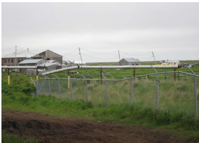
Photo 9: Break in Pipeline from Washeteria to Sewage Lagoon
