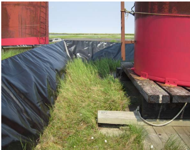
Photo 5: Secondary Containment around NVC Tank Farm
