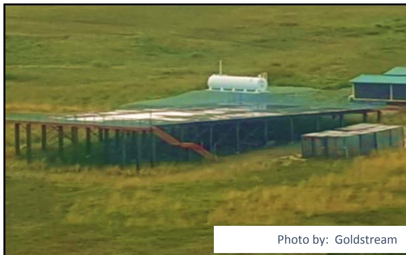
Figure 10: 5,000-Gallon Double-Wall Tank Near MEC Foundation
