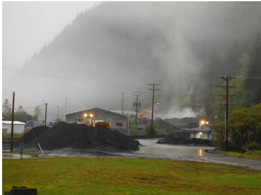
Figure 5-12 Lowell Creek Bridge Covered - 9/20/2012 (URS 2012)
