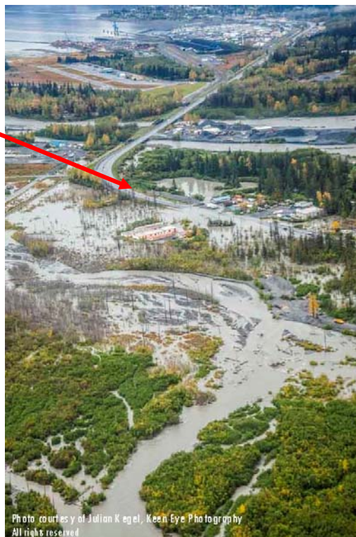
Figure 5-13 Seward Highway Flooding (SBCFSA 2012)
