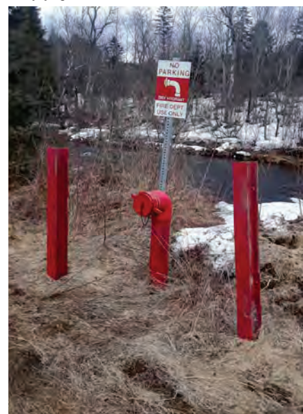
Dry Fire Hydrant in East Haven, Vermont. Source: Artaxerxes
