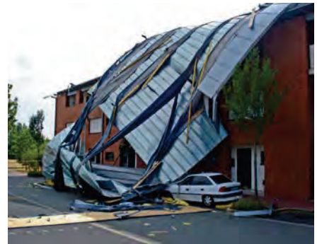
Exhibit 5-78. Wind Damage to Roof
