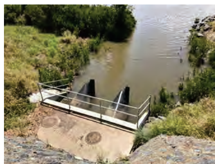
Exhibit 5-69. Backflow Device Prevents Stormwater Flooding in Australia
