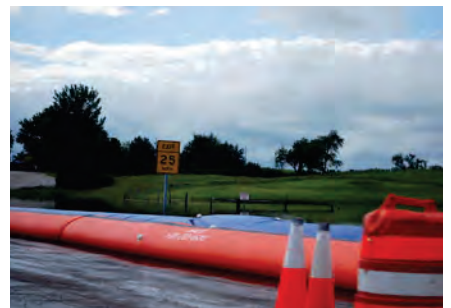
Exhibit 5-77. Deployable Flood Wall
