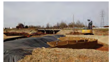
Exhibit 5-44. Soil and Stream Protection During Construction
