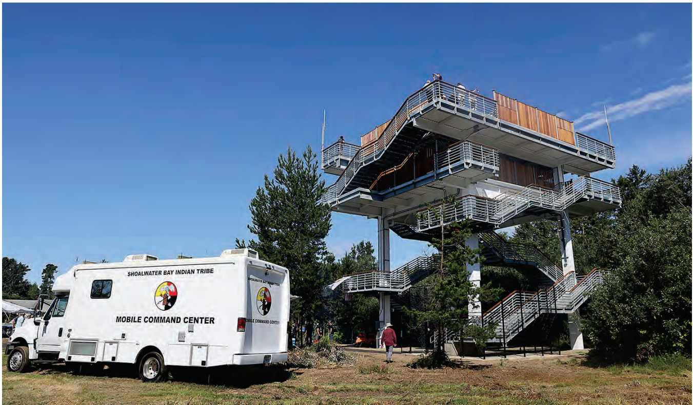
A vertical evacuation structure built to protect the Shoalwater Bay Indian Tribe from tsunami effects in Washington State. Source: Washington Military Department, https://mil.wa.gov/news/celebrating-nations-first-tsunami-vertical-evacuation-tower
