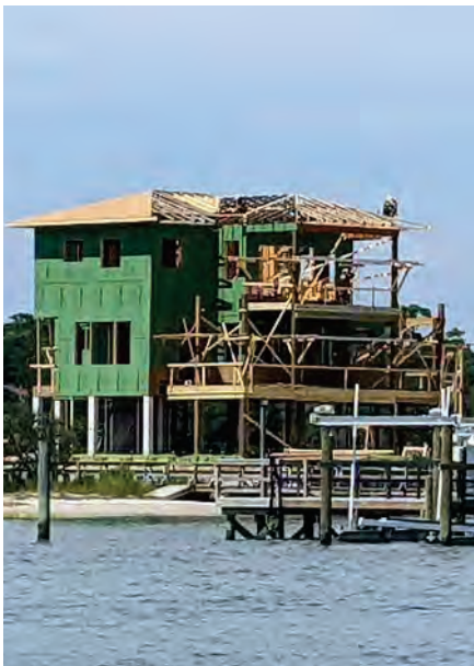
Exhibit 5-74. Coastal Home Elevated on Piles Under Construction, Wilmington, North Carolina
