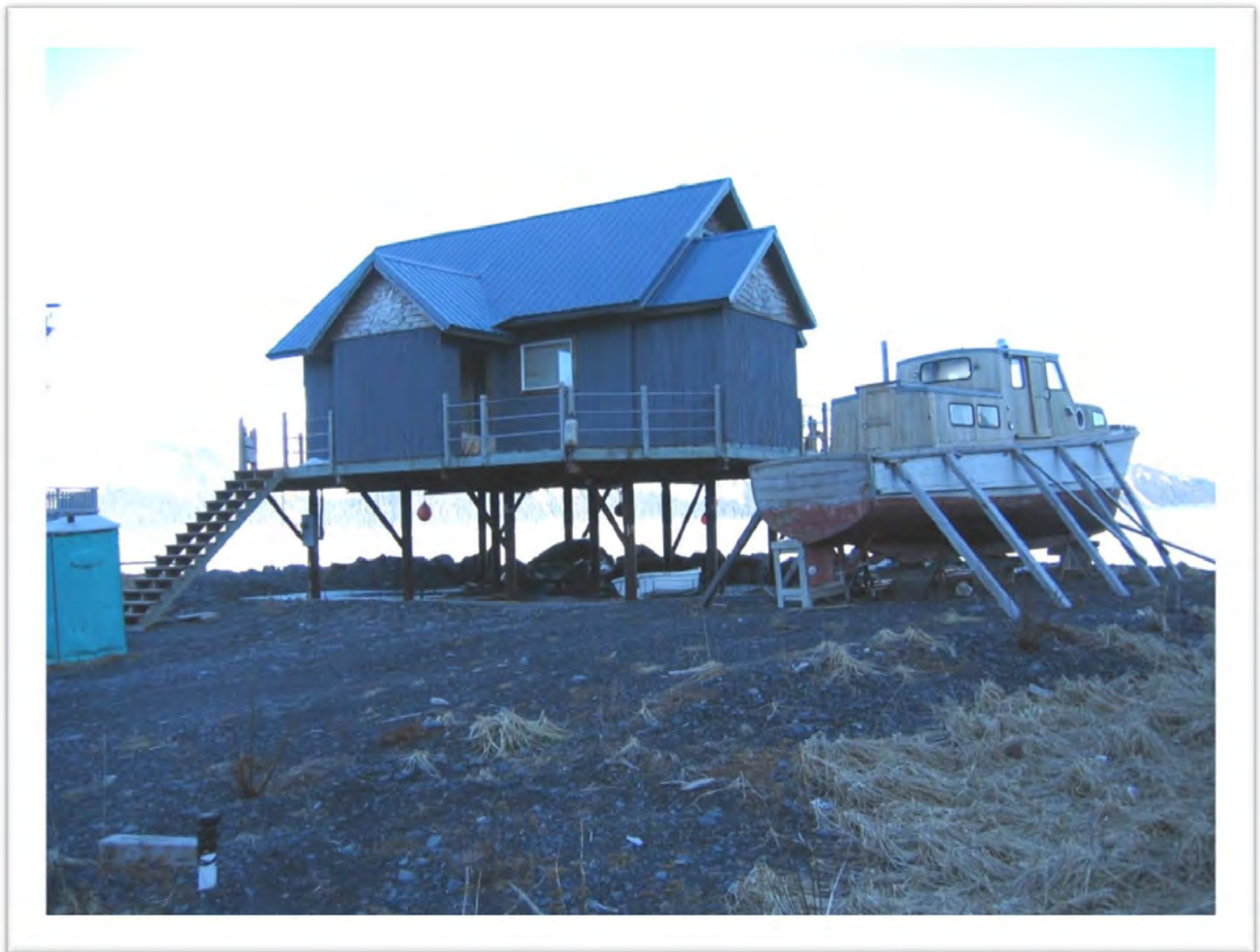
Figure 3: Tsunami and Coastal Flood-Elevated Home, Lowell Point, Kenai Peninsula Borough
