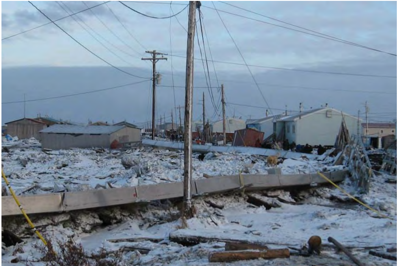
Figure 7: Storm damage in the Village of Kotlik, Alaska, November 2013
