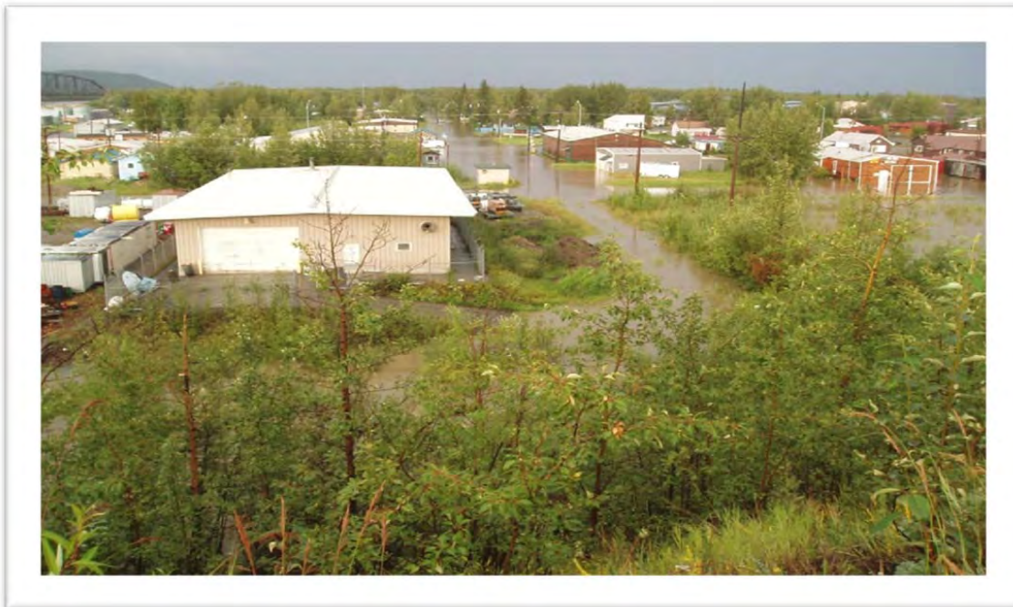
Figure 16: City of Nenana, 2008 Flood
