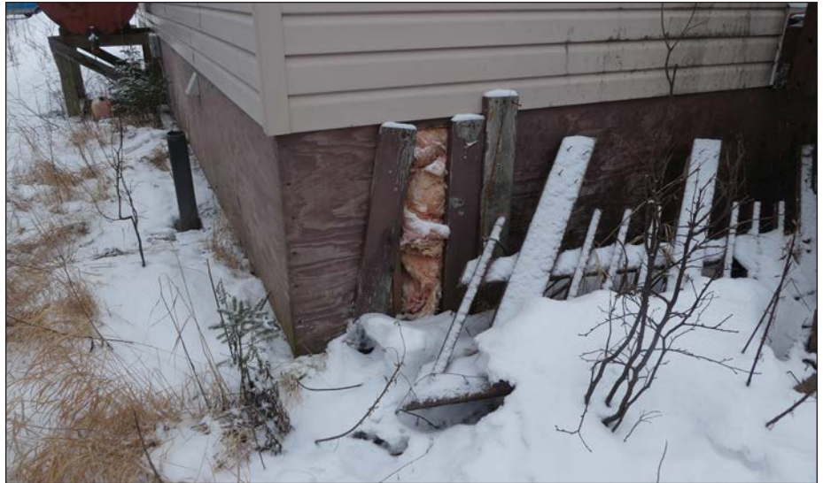
A visual inspection of the building exterior should be done to document any damage to the structure, such as damaged roofing or siding.
