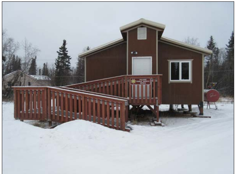
The VPSO office is in good condition and is mainly used when there is an occupant in the holding cell.
