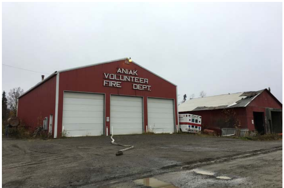
The fire station could reduce energy costs by employing its waste oil and cordwood boilers instead of the fuel-oil-fired boiler.
