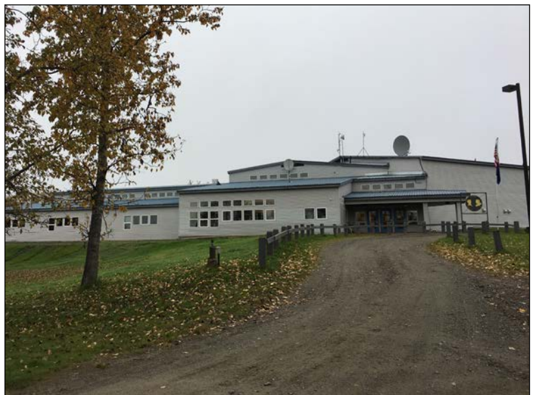
The school could reduce its energy costs by $15,000 through an energy retrofit.
