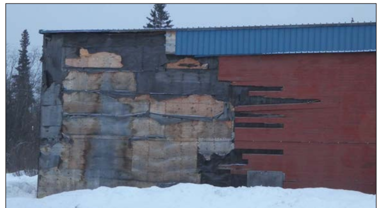
Look for and document any damage to the structure, such as damaged roofing or siding in a monthly inspection of the building's exterior.
