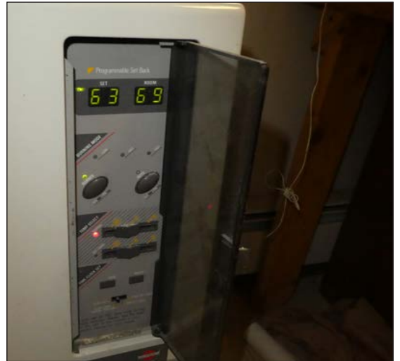
The Toyotomi stoves should be checked on monthly to ensure that the programmable thermostat is set at 63°F in the winter during unoccupied times.
