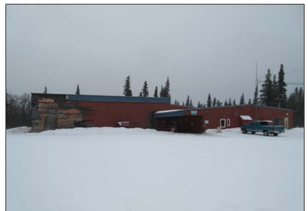
The community center building is in poor condition but continues to host social events and house laundry facilities.
