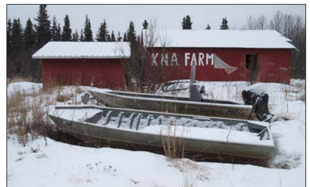
The small farm building is in poor condition and is currently serving as a cold storage facility.
