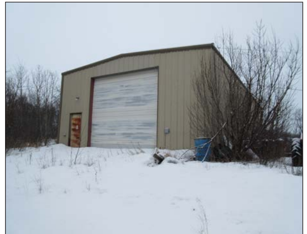
The large farm building is in poor condition and is currently serving as a cold storage facility.
