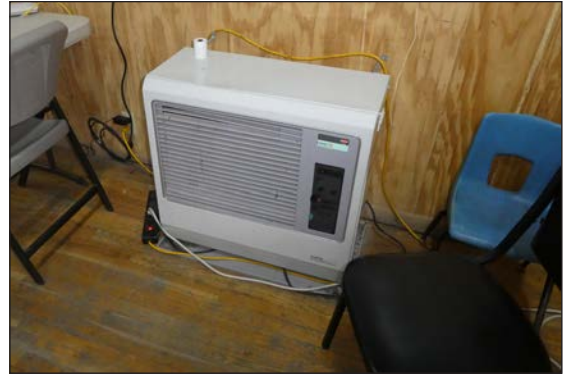
The Monitor and Toyotomi stoves should be checked monthly to ensure that the programmable thermostats are running correctly.
