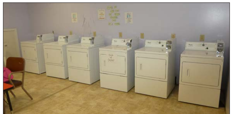
The laundry equipment should be checked each month to make sure they are working properly.
