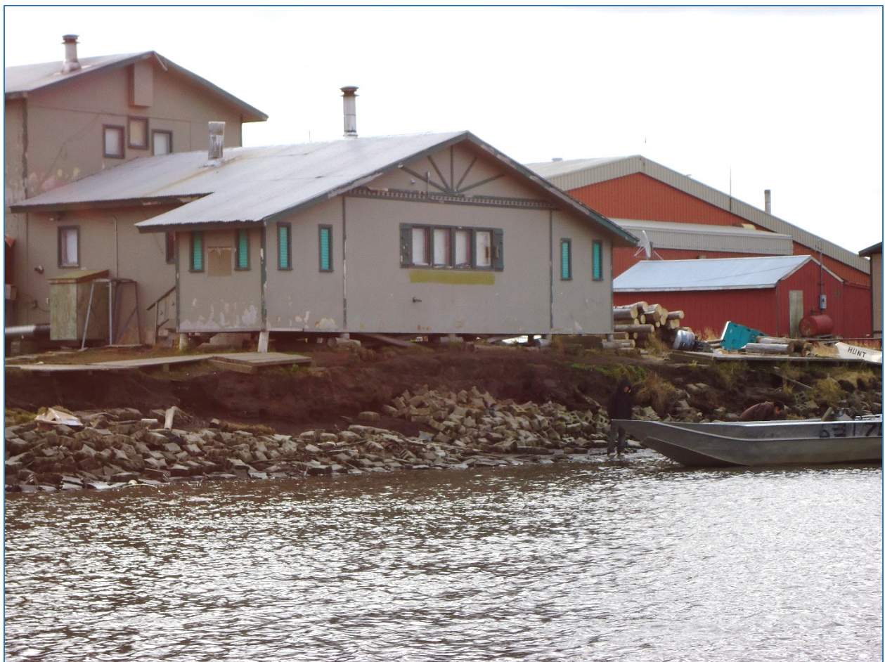
Figure 6: Erosion of the Kotlik River Bank in 2011. Photo: DCRA Photo Library
