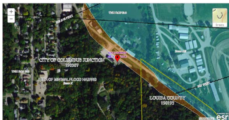
Figure 14. The new water treatment plant in Columbus Junction, Iowa.
