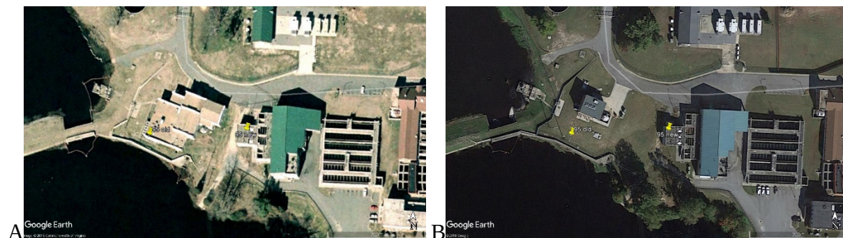
Figure 11. Portsmouth's water treatment plant: A) in 2003, and B) in 2015.
