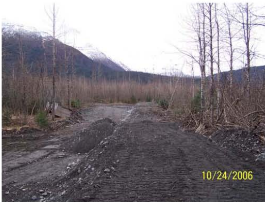
285' dike at the end of the airstrip.
