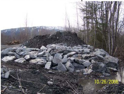
Rip rap on the 130' extension.
