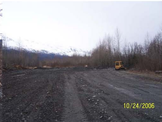
130' extension to existing dike.
