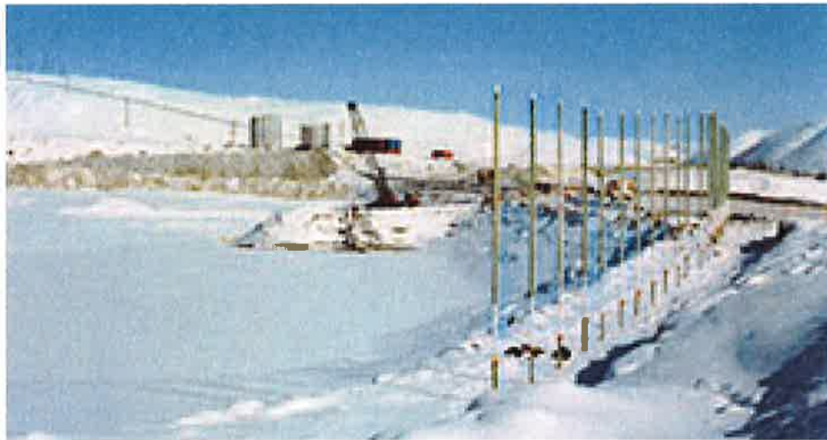
Photo of thermosiphon dam at the Kubaka Gold Mine; Russia Far East
