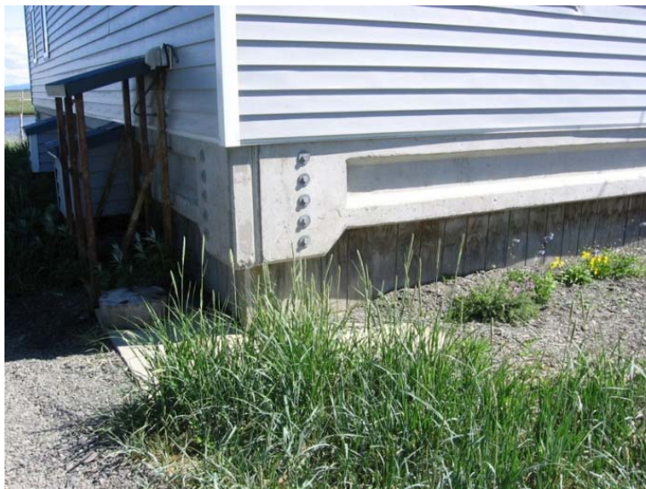
Figure 5 - New structure with elevated, pre-cast concrete foundation
