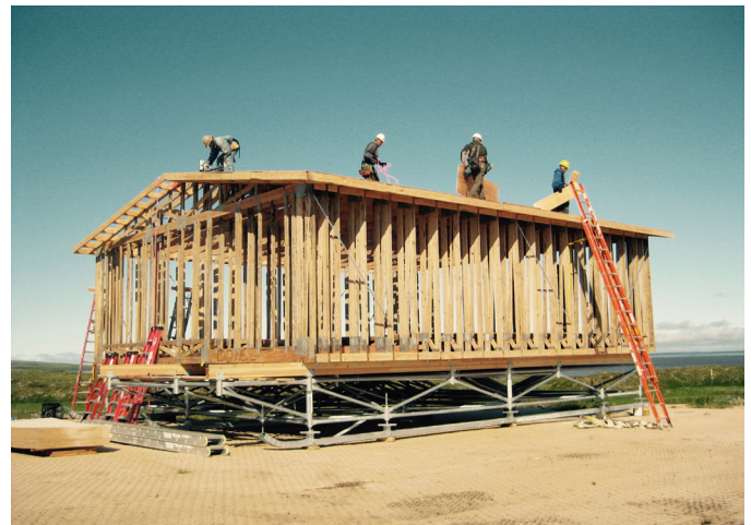
Above: The crew framed out the entire integrated truss structure in 1.5 days.
