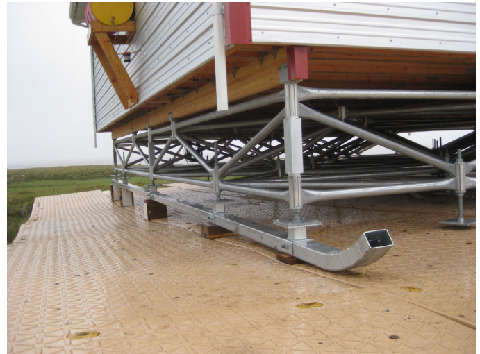
Above: The Triodetic foundation in the Demonstration Home allows for adjustability should differential movement in the frost layer or permafrost affect the home. The skids allow the building to be moved from the Bivouac Site to the home's final plat after construction.
