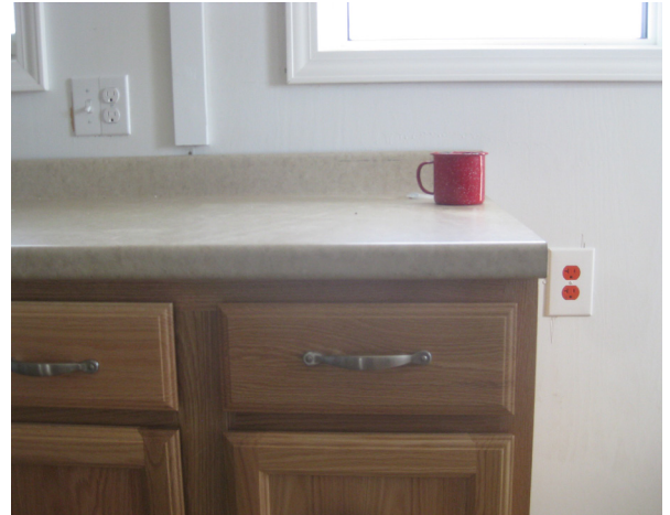
Above: Color-coded outlets in the Demonstration Home allow the occupant to know which outlets work when the house is on battery power.
