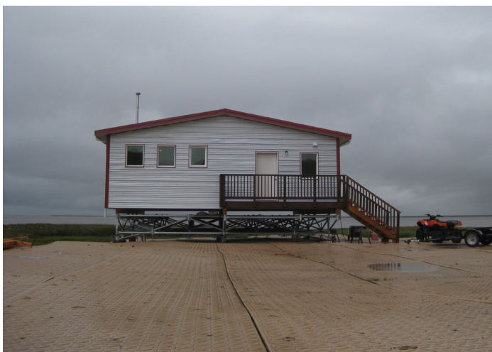
Above: The CCHRC Mertarvik Demonstration Home was built at the former IRT Bivouac Site in 2016. The Bivouac Site has enough room for approximately five more homes of this size to be efficiently constructed. The homes could then be moved to their final site/plat.
