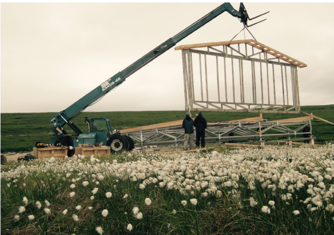
Above: Integrated Trusses greatly speed up construction time during a short season. Here a squirt boom was used to raise the trusses.
