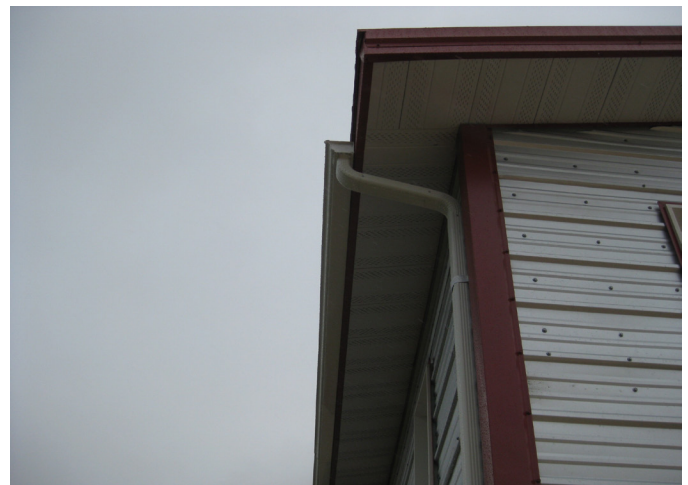
Above: Durable cladding such as ribbed metal sheathing will stand the test of time while minimizing maintenance, repainting, or water damage over time.
