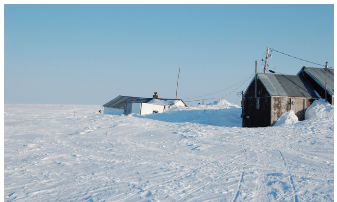
Above: The same house as at left in later winter. The home has been almost completely buried due to wind drift action.
