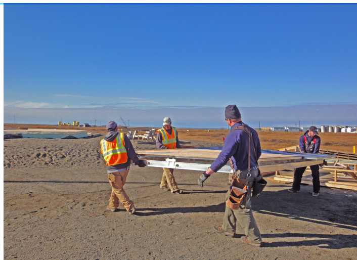
Above: The sections of wall are light enough for four workers to carry. The wall system can be prefabricated inside a shop during the off-season or inclement weather and carried to the site during construction.
