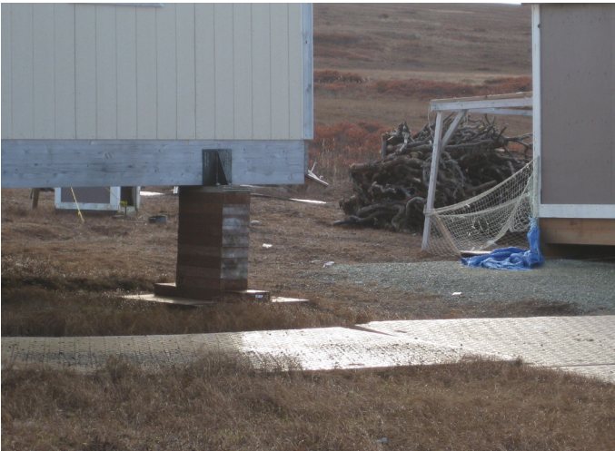
Above: At the homes near the MEC, dunnage posts rest directly on an oversize footing. This type of foundation is potentially unstable.
