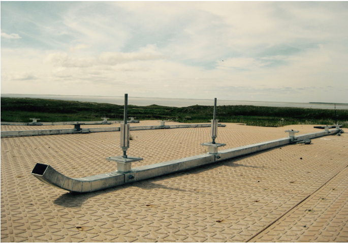
Above: Until plats and pads have been developed, homes at the new site can incorporate ski-shaped footings to enable movement from the staging area.
