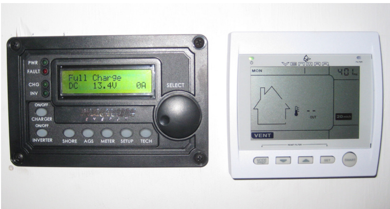
Above: The control panels for the electric system and the ventilation system are adjacent to each other in the main living space, giving occupant control to both systems.
