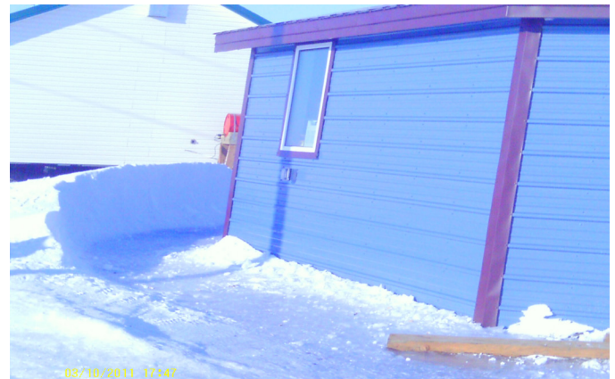
Above: An octagonal prototype in Quinhagak with an on-ground foundation. The geometry of the home self-scours wind born snow to prevent drifting.
