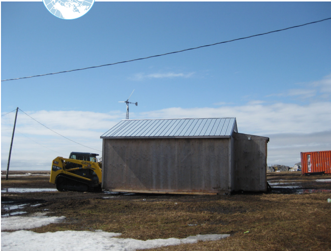
Above: At the Newtok Site, a building is moved on skids at Breakup to a new location in the village using a small dozer.
