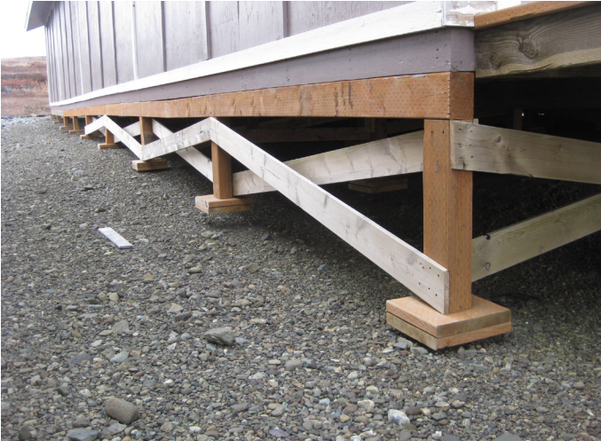
Above: There has been significant movement in this pad. The IRT shed foundations are not adjustable.
