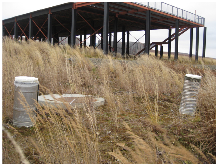
Above: The septic and drainfield for the Mertarvik Evacuation Center is already in place, and may be a resource for waste disposal during the transitional phase.
