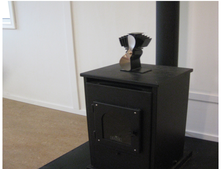
Above: An oil-drip stove allows for heat without needing electricity, an important feature in the first pioneer homes built before the grid.
