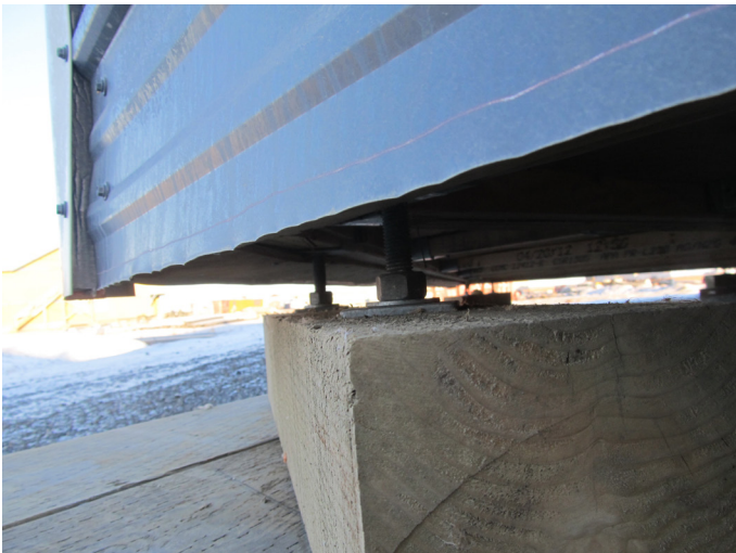
Above: An adjustable foundation on cribbing in the village of Quinhagak. This home can be adjusted to account for movement of the ground over time.
