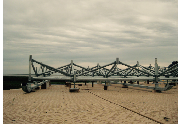
Above: Triodetic foundations allow for adjustability should differential movement in the permafrost affect the home.
