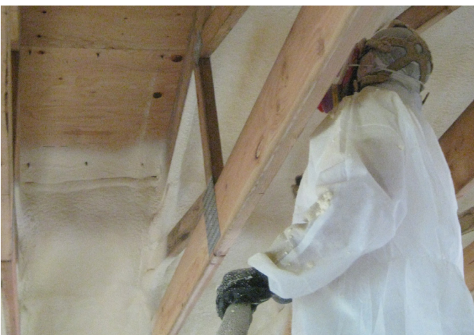
Above: Spray-applied polyurethane insulation creates a monolithic thermal envelope and also functions as a vapor retarder in the home, creating an extremely warm building envelope that requires ventilation.
