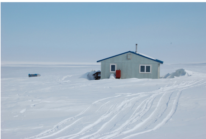
Above: A home at the Mertarvik site in early winter. Snow drifting has already begun to accumulate. Snow drift will need to be considered carefully in the layout of adjacent houses and shape of new housing to ensure that the drifting issues of Newtok are not a problem in Mertarvik.
