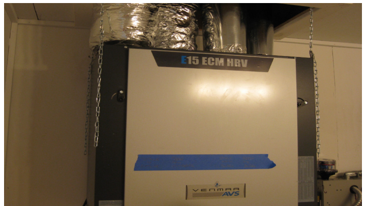
Above: Heat Recovery Ventilation saves energy by preheating incoming air while ensuring safe and healthy indoor air quality in the home.
