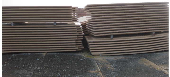
Above: A significant amount of Durabase road material has been stockpiled at the staging area, along with steel dowels and cap pieces for assembly.
