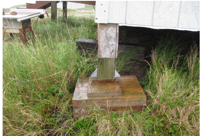
Above: At the original houses near the spring at Mertarvik, post and pad foundations rest directly on the ground.
