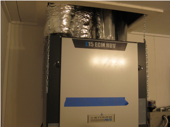
Above: The Heat Recovery Ventilator preheats fresh intake air before distributing it to the household.
