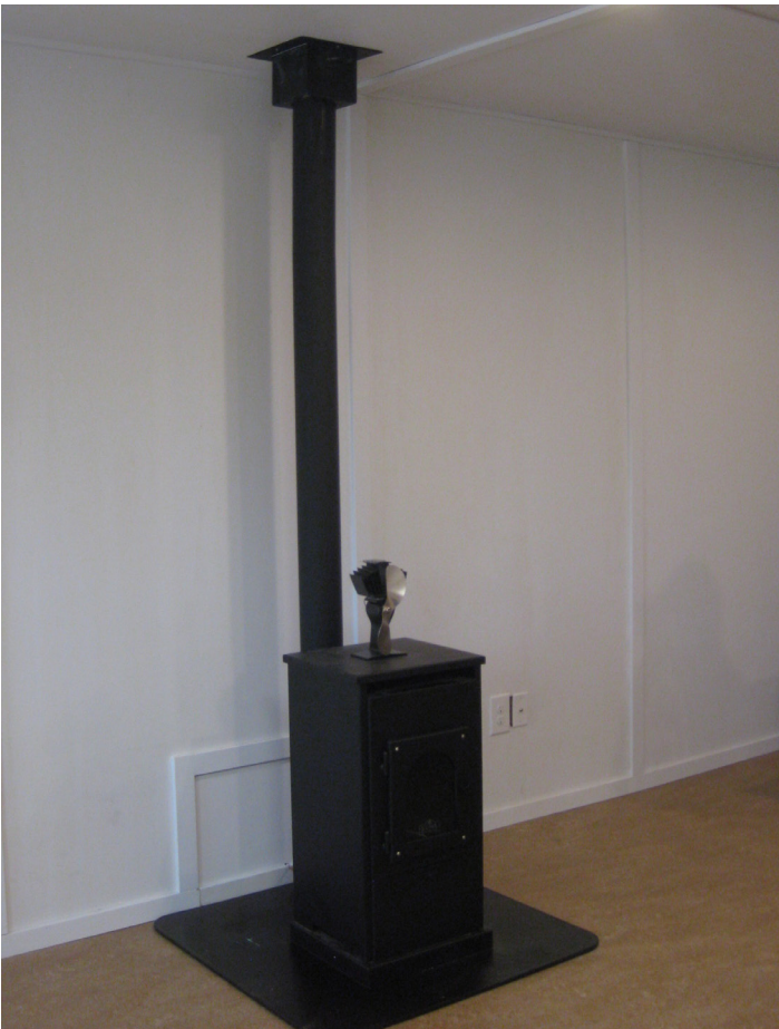
Above: The Demonstration Home in Mertarvik uses an oil drip stove, which does not require electricity to heat the home. Once electrical infrastructure is present in the village, homes may use the more common monitor or Toyotomi heating appliances.
