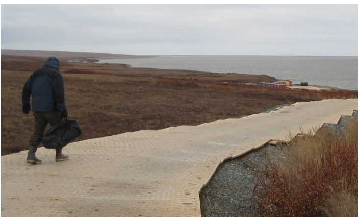
Above: The Durabase road from the MEC site, looking downhill toward the staging area and barge landing.
