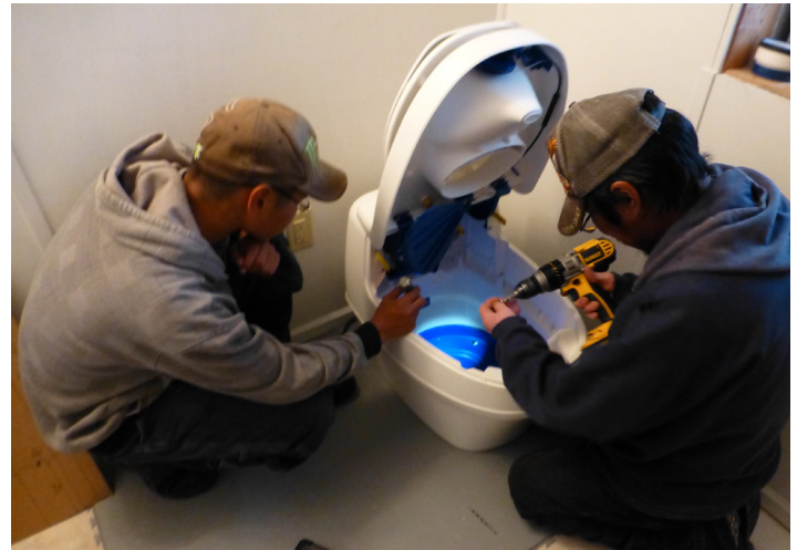
Above: Residents of Atmautluak install a separating toilet in a prototype home.
