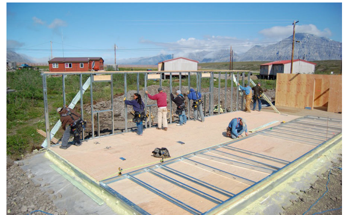
Above: CCHRC has also designed and constructed foam "floating foundations", which span variations in the pad below it, should changes in the thermal regime of the soil cause settlement. The foundation can also be jacked with structural foam back to level if necessary.
