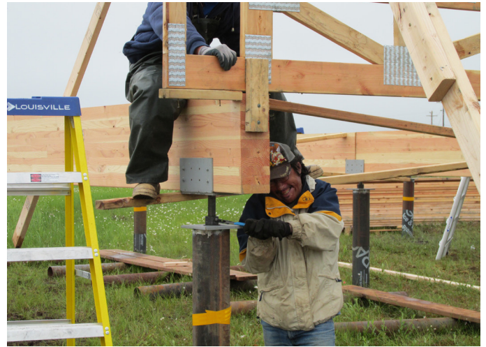
Above: An adjustable pile foundation under construction in the village of Atmautluak. A cheater bar was later welded onto the wrench for periodic releveling of the foundation.
