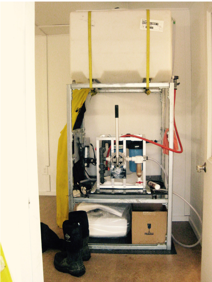
Above: The water treatment plant in the Mertarvik Demonstration Home.
