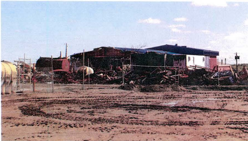
LKSD workers are preparing the Kilbuck fire debris for cleanup.
