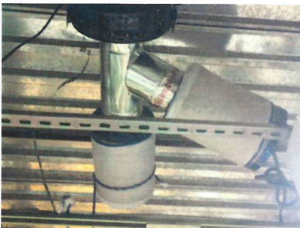
Double 6" x 16", 400 CFM activated carbon canisters – Vegetation Room
