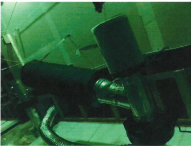
Active Air 8" x 39", 950 CFM activated carbon filter and 6" x 16", 400 CFM activated carbon canister – Flower Room B
