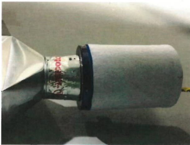
6" x 16", 400 CFM activated carbon canister – Reservoir Room
