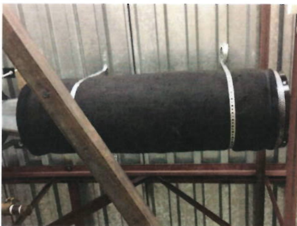
Active Air 8" x 39", 950 CFM activated carbon filter – Flower Room C
