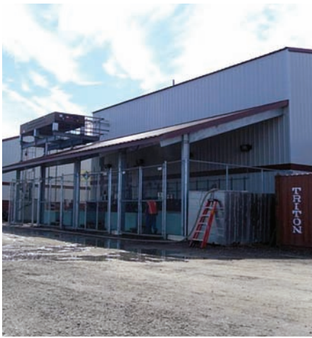
NSSC's cold storage facility in Nome opened for operations in June 2009.
