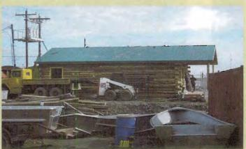
In 2009 Kwikpak Fisheries constructed a building out of logs which were collected as they drifted down the river. The logs were cut at the Emmonak sawmill throughout the winter. This building will be used in 2010 to house the fishermen's store.
